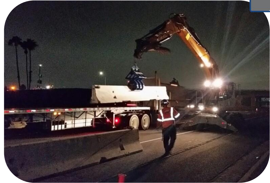
Placing k-rail
