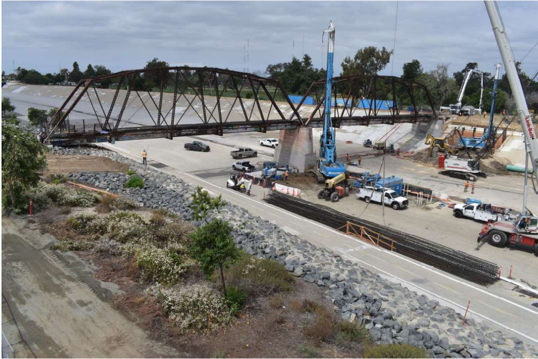
Photo taken 6/26/19 looking southwest
