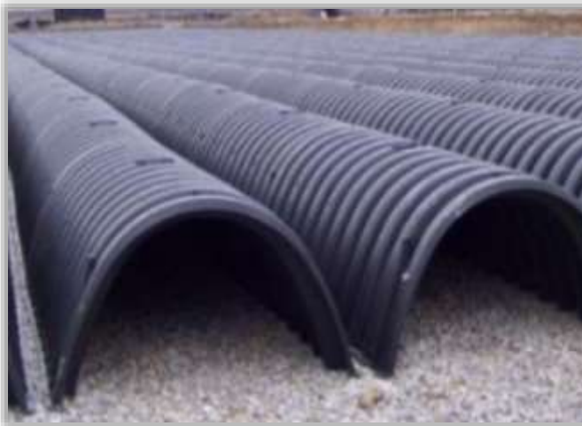
Underground Infiltration / Infiltration Gallery
