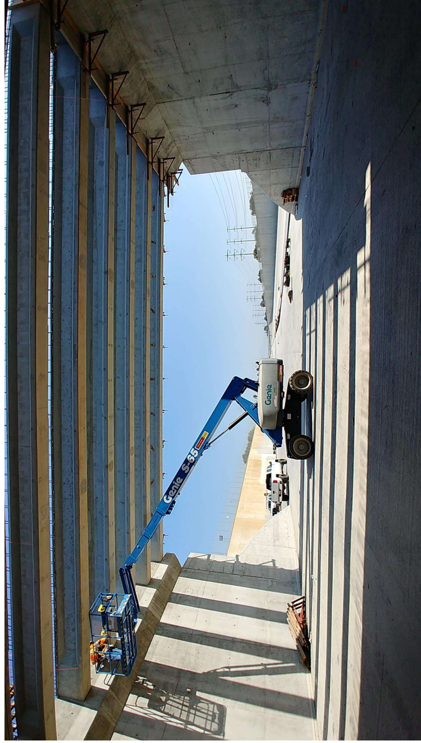
Santa Ana River bridge construction
