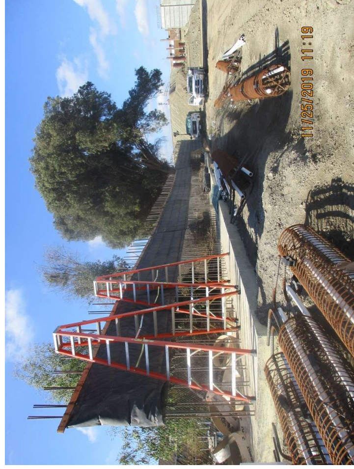
Retaining wall and soundwall construction
