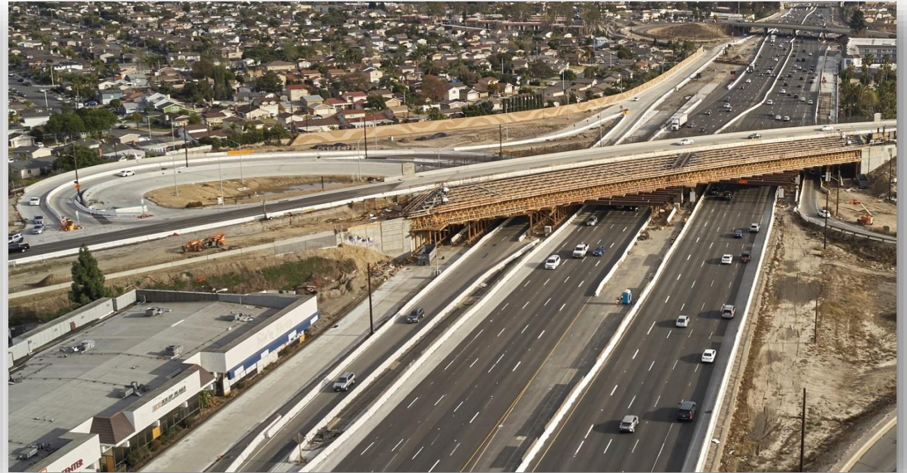
Magnolia Street bridge construction
