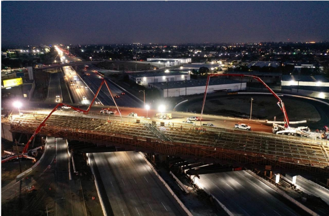
Bolsa Avenue bridge construction
