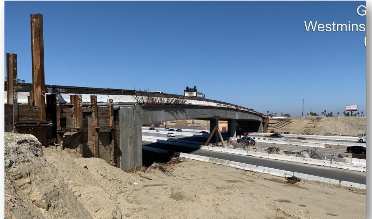
Goldenwest Street bridge construction
