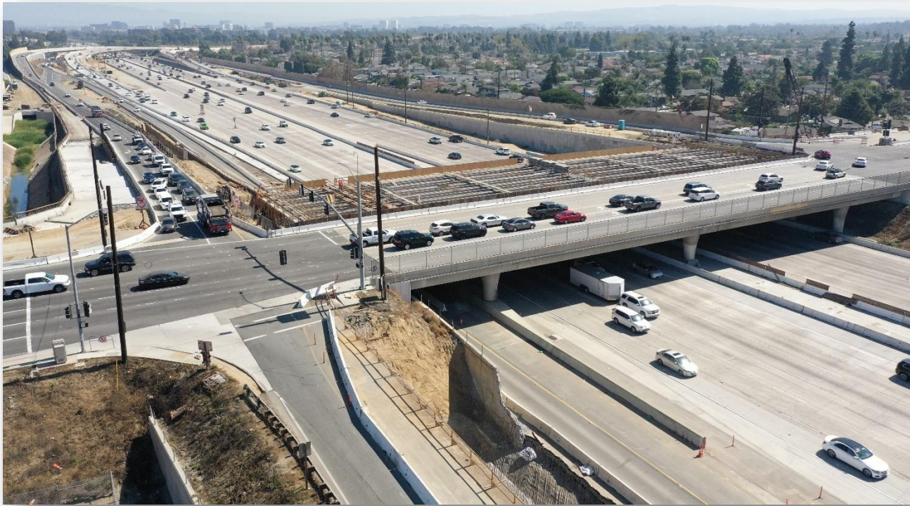
Fairview Road bridge construction
