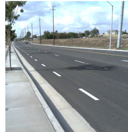
Bastanchury Road Improvements City of Yorba Linda
