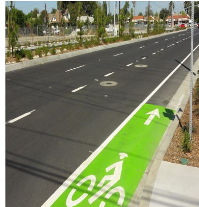
Grand Avenue Improvements City of Santa Ana
