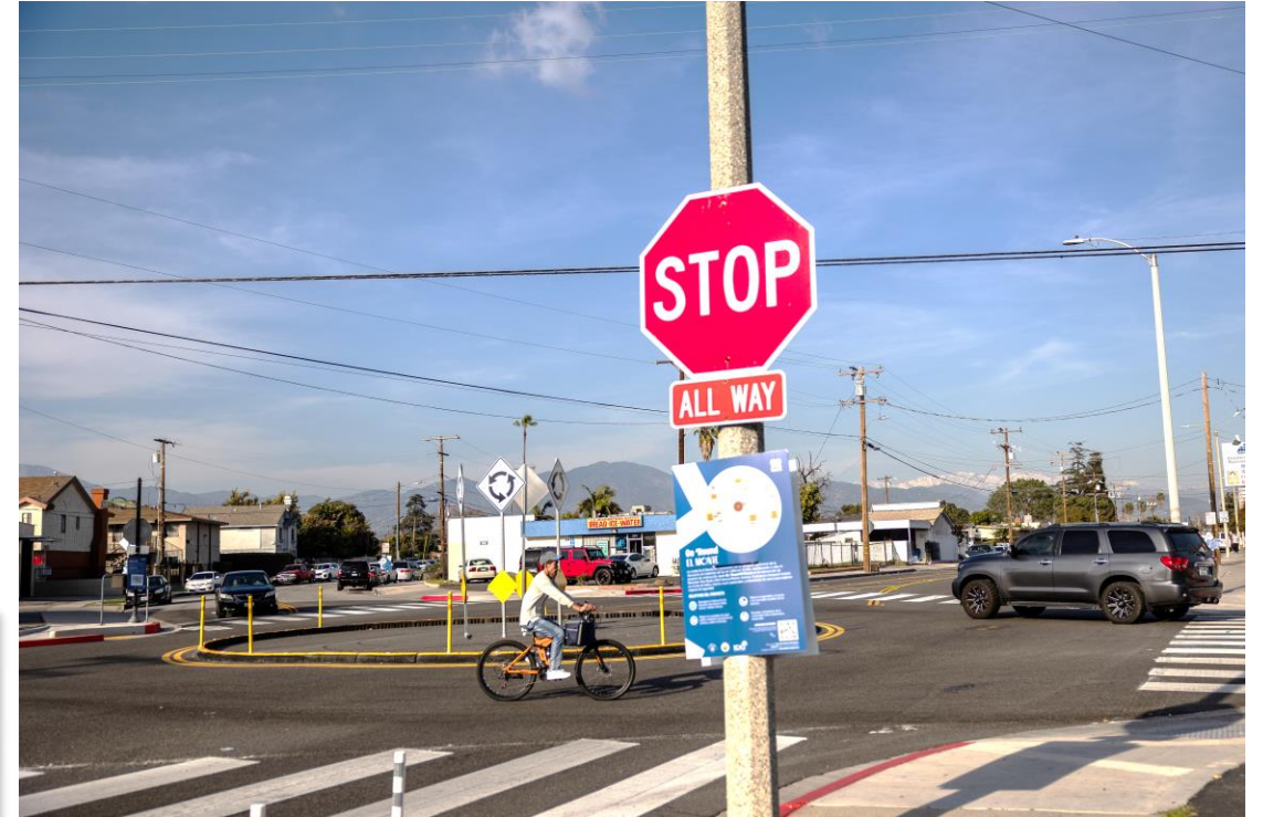
Mountain View Road, After
