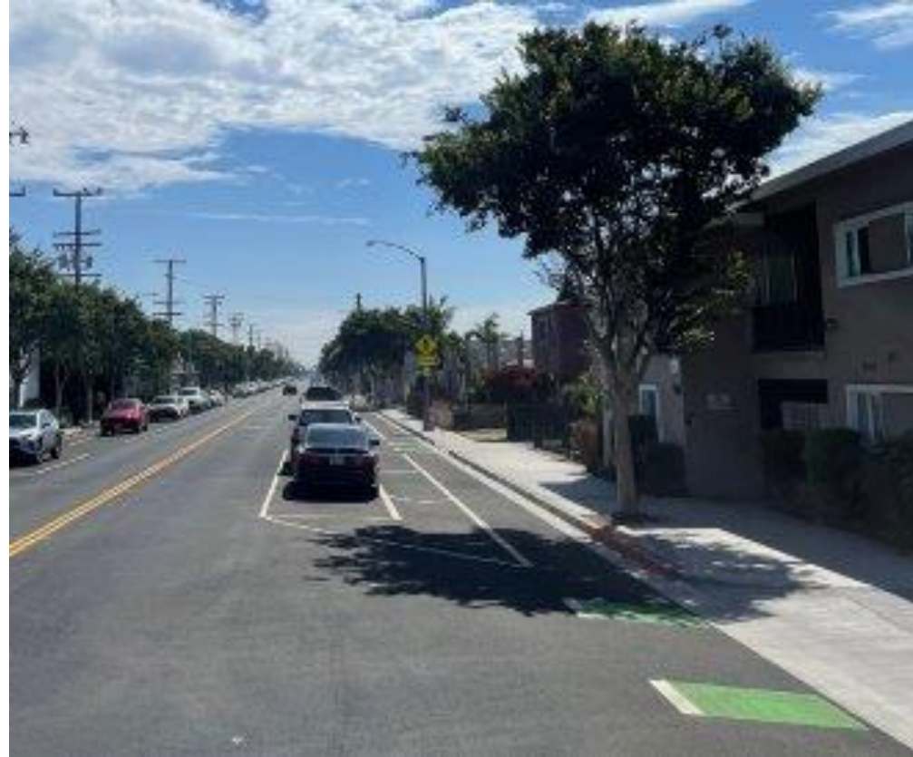
South Street, After
