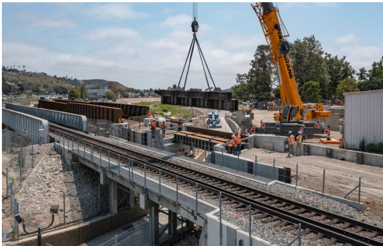
Crews erecting steel girders above the bike path.
