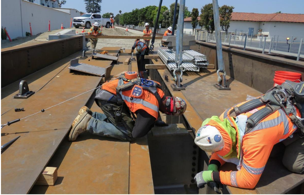
Crews connecting two girder assemblies
