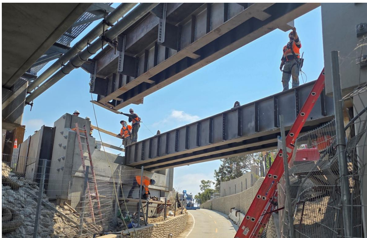
A second girder is being positioned above the bike path
