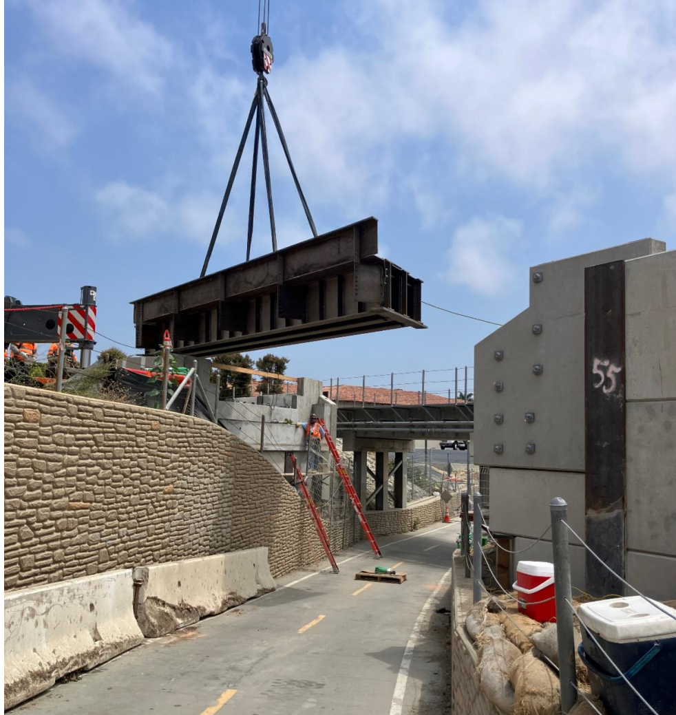
Steel girder being hoisted into place
