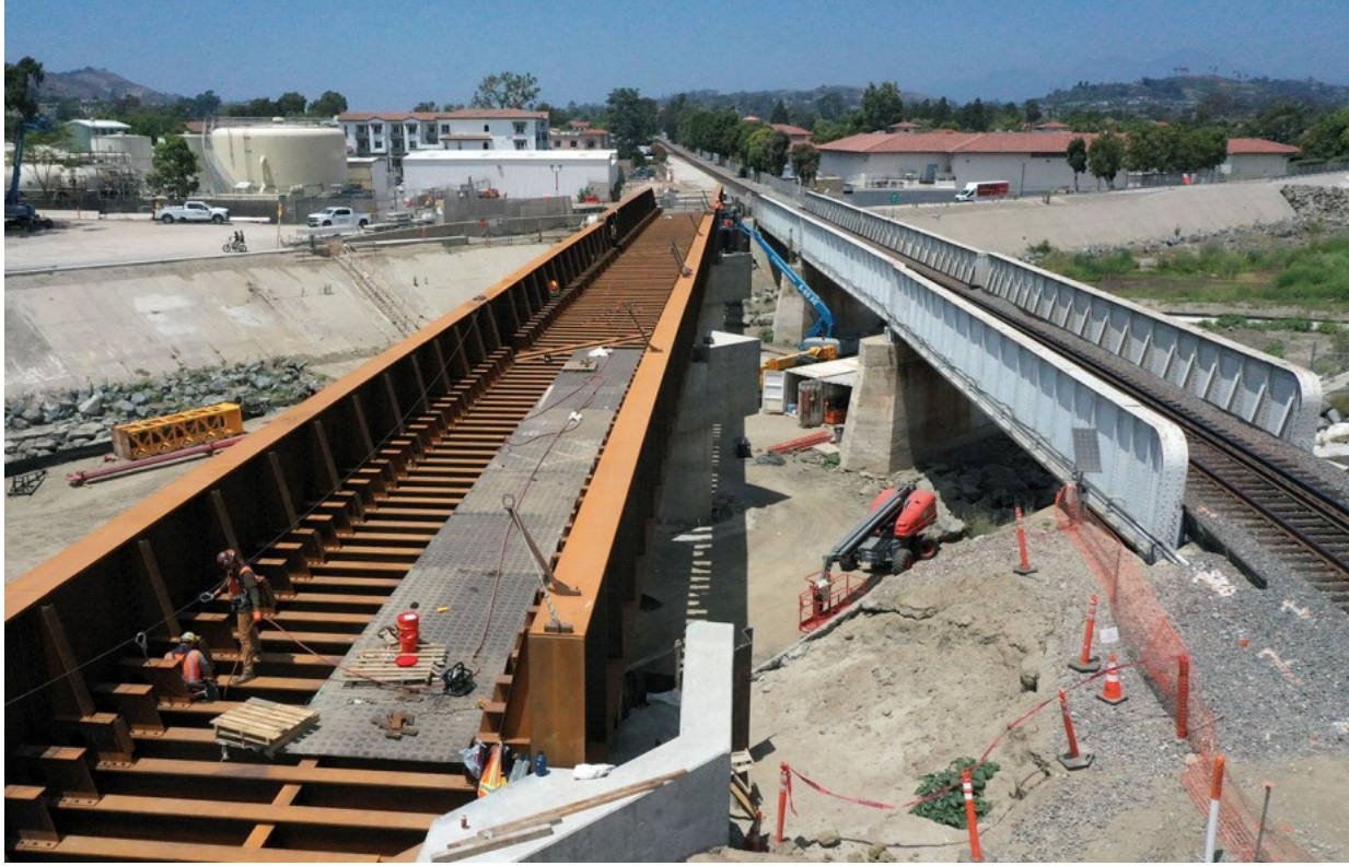
Crews constructing the main steel bridge spans
