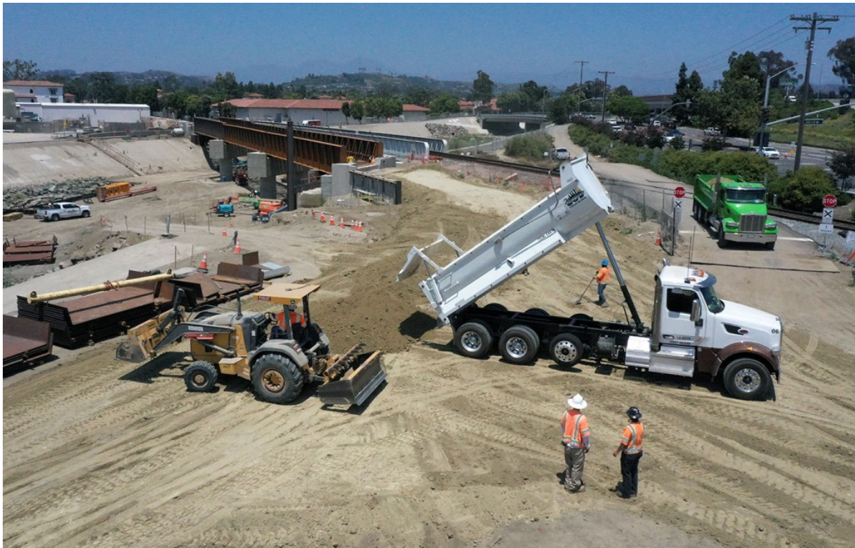
Crews delivering embankment fill material
