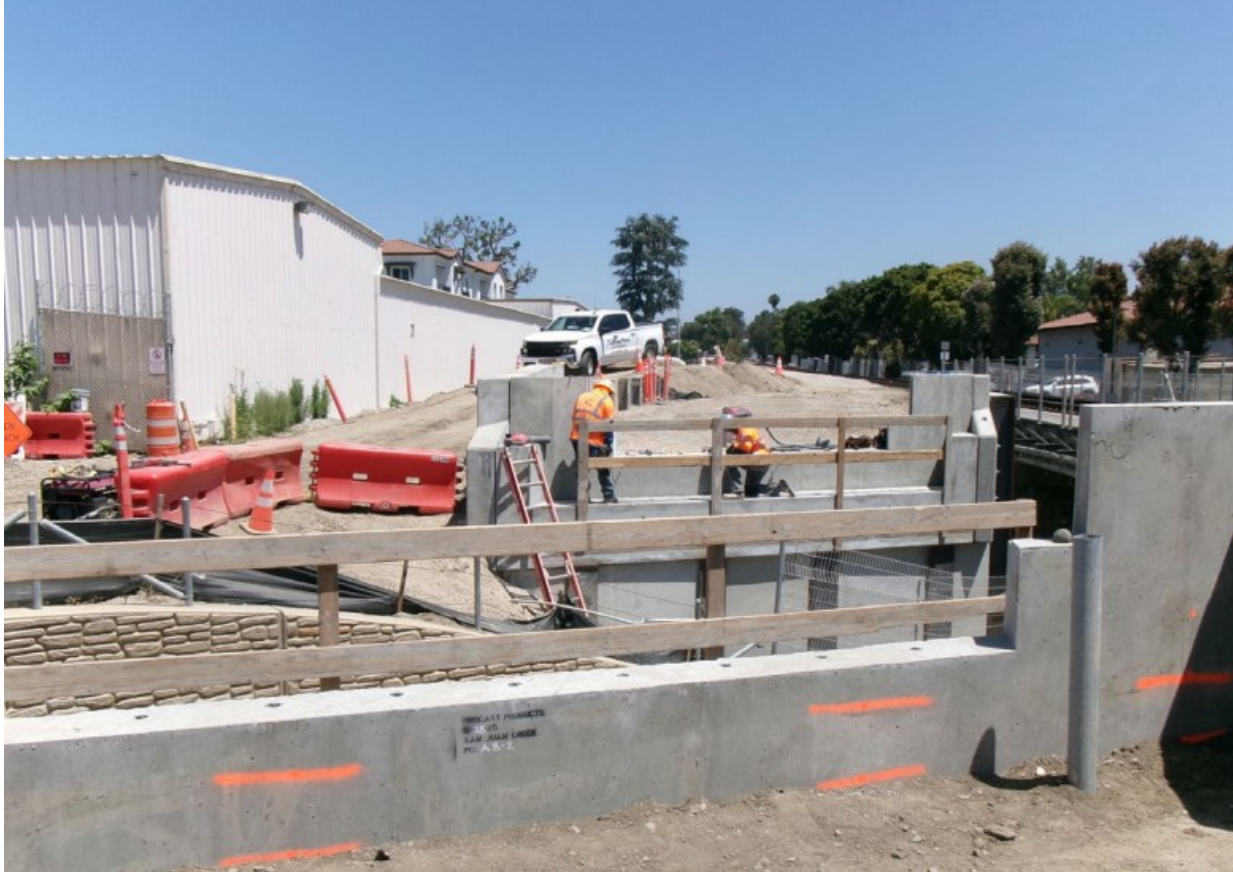
Abutment construction to support the bridge above the San Juan Creek Trail
