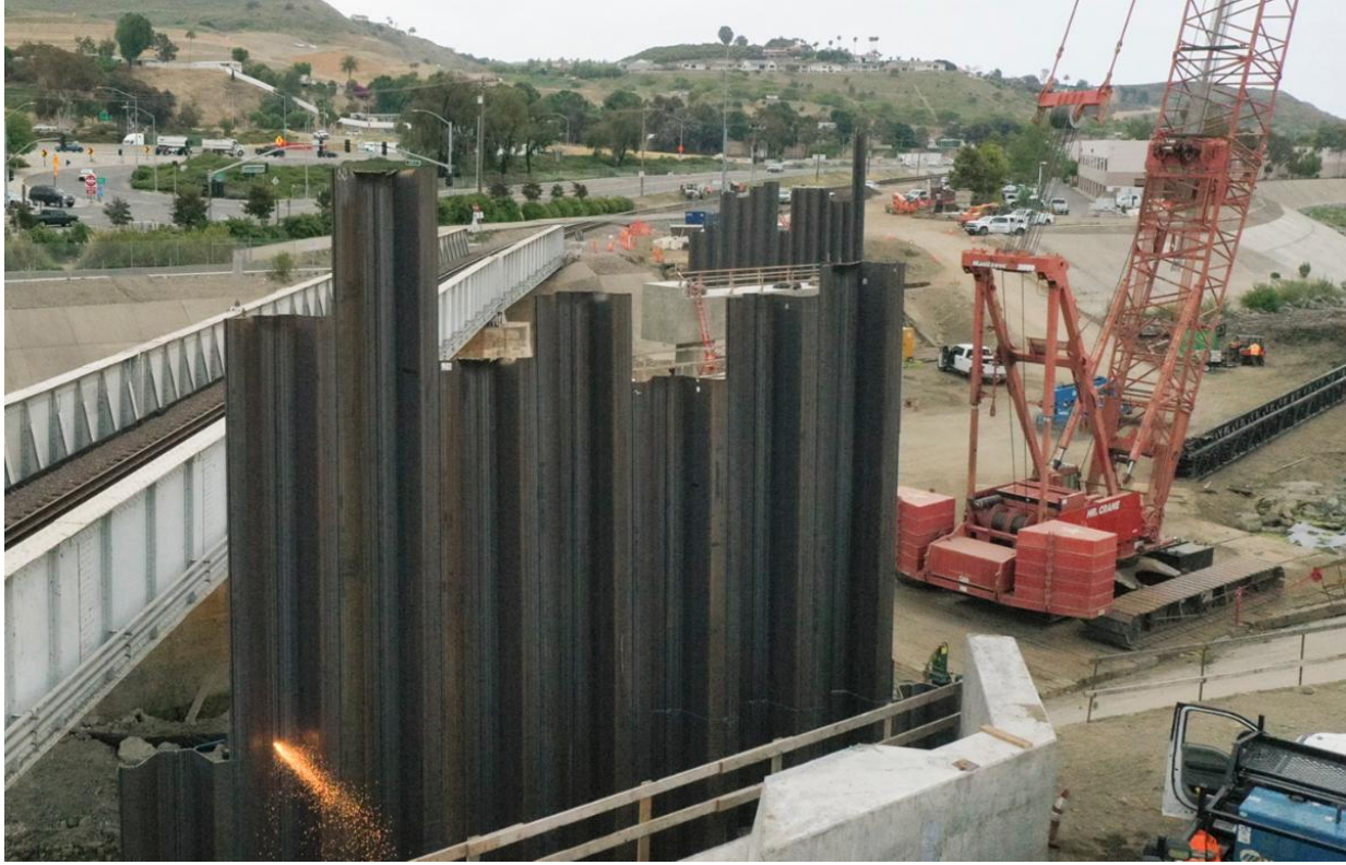
Crews torch cutting sheet piles.
