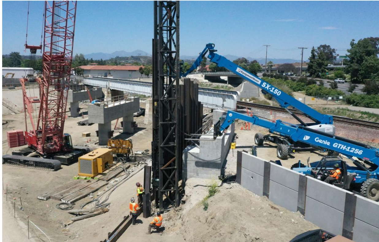
Crews installing sheet piles.
