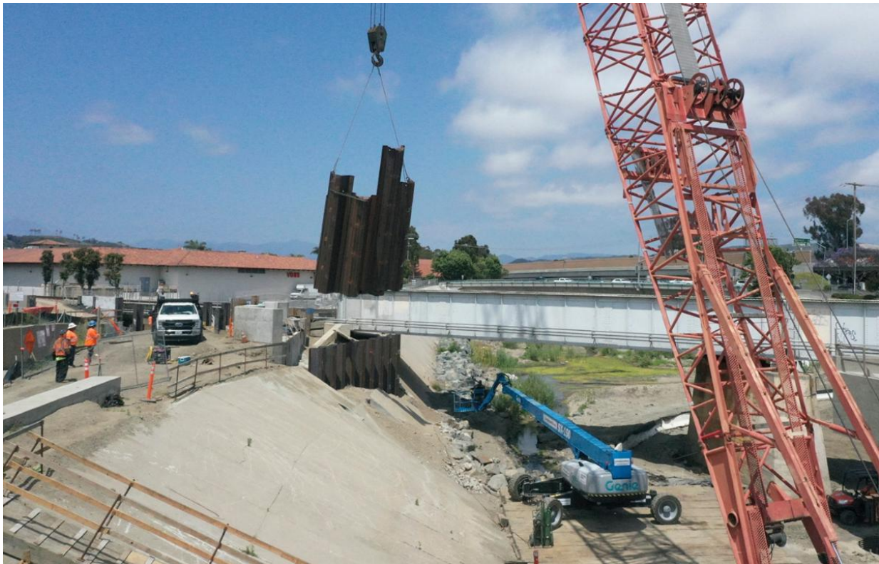
Crews hoisting sheet piles parts that were cut off.
