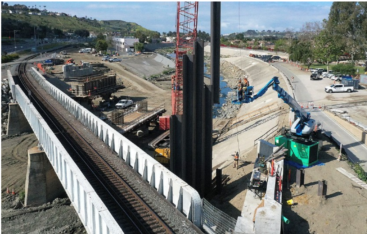
Crews installing sheet piles.
