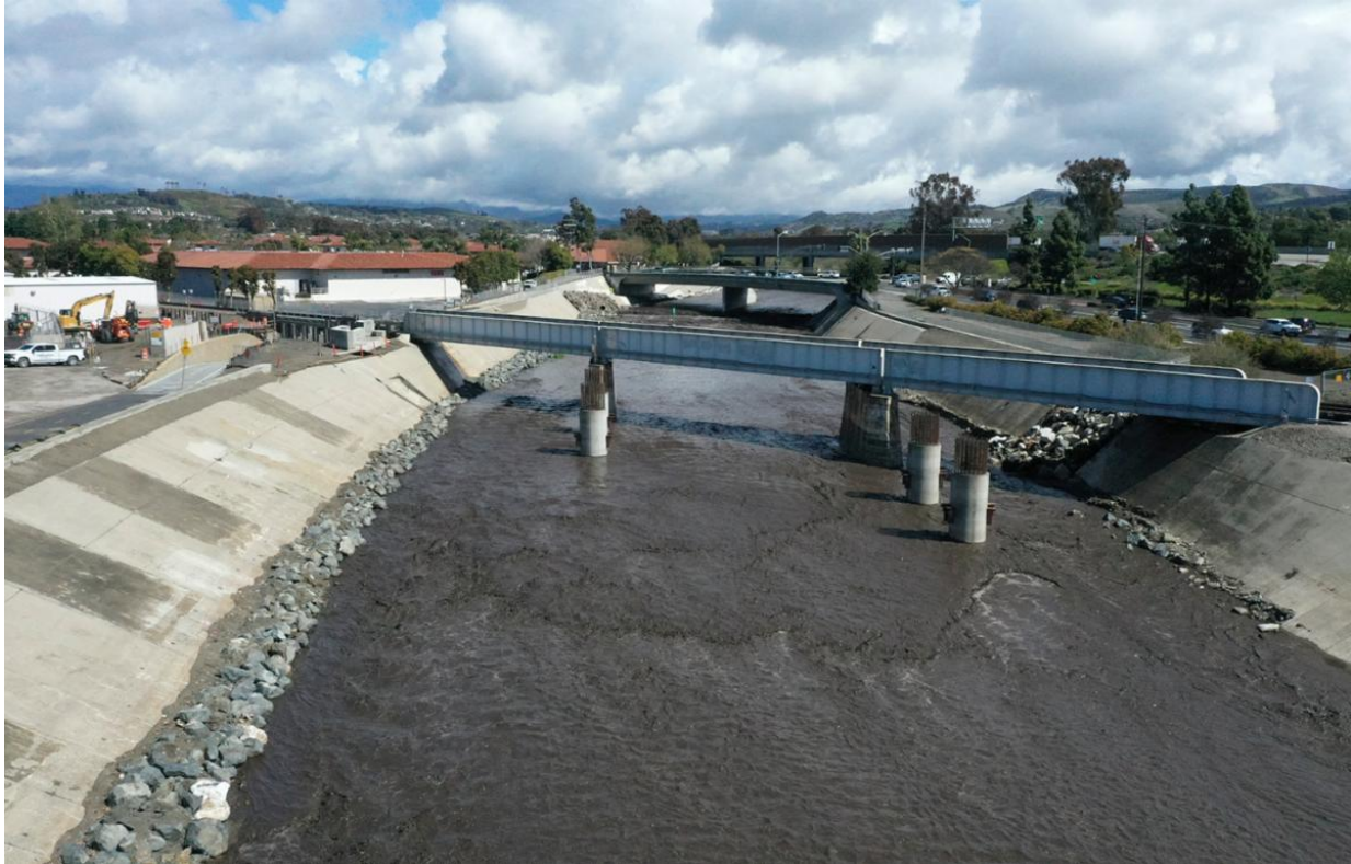
New railroad bridge foundation structures installed last year.
