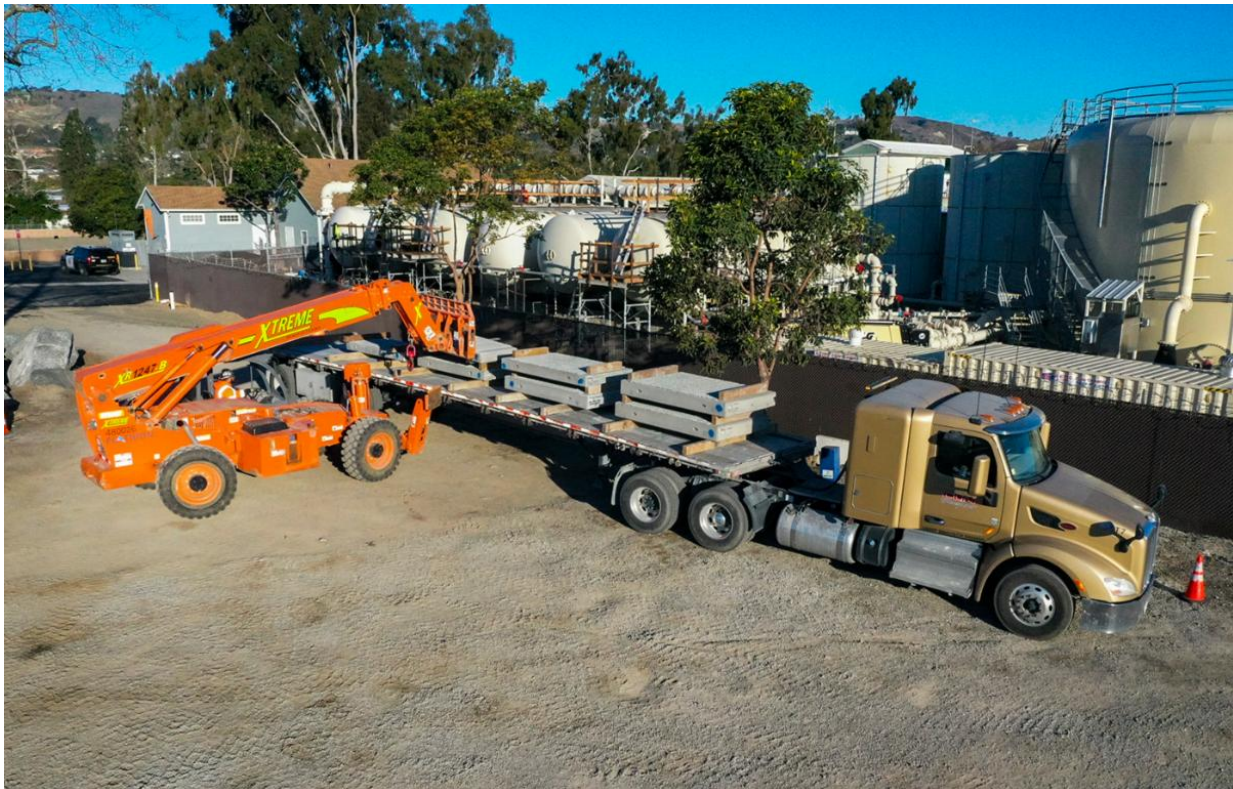
Retaining wall panels being delivered to the construction site.
