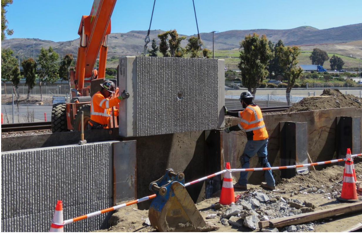
Crews installing retaining wall panels.
