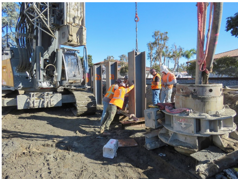
Steel pile installation for one of four retaining walls.
