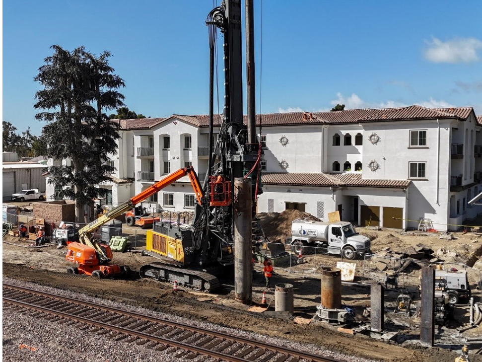
Drilling operations for retaining wall pile installation.
