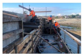
Crews constructing abutment "formwork" to prepare for concrete pours.
