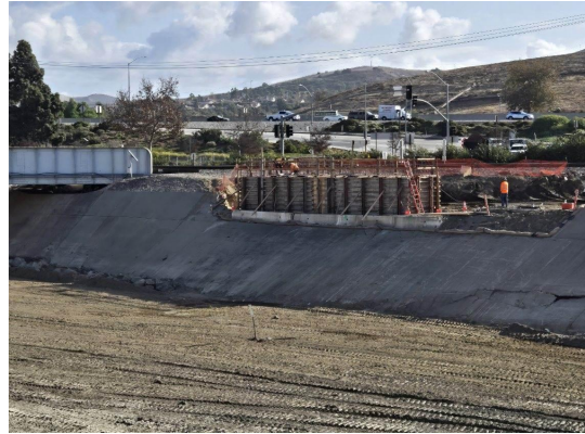
Retaining wall construction
