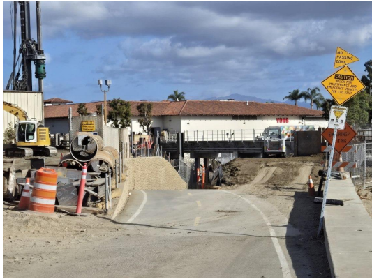
Crews continue working on San Juan Creek Bridge
