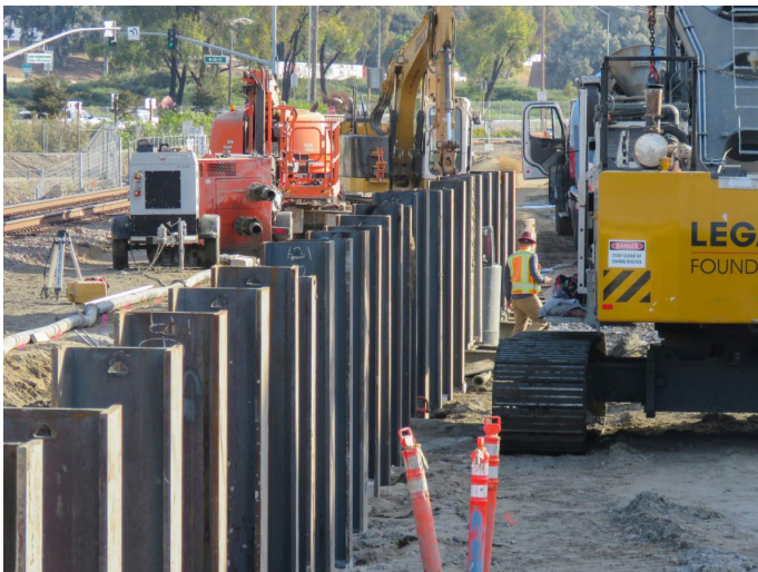
Retaining wall construction.
