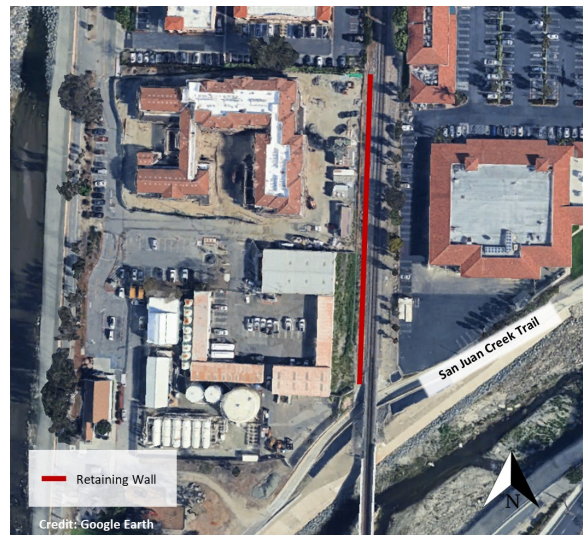
Aerial view showing the location of a new soldier pile wall that is being constructed.
