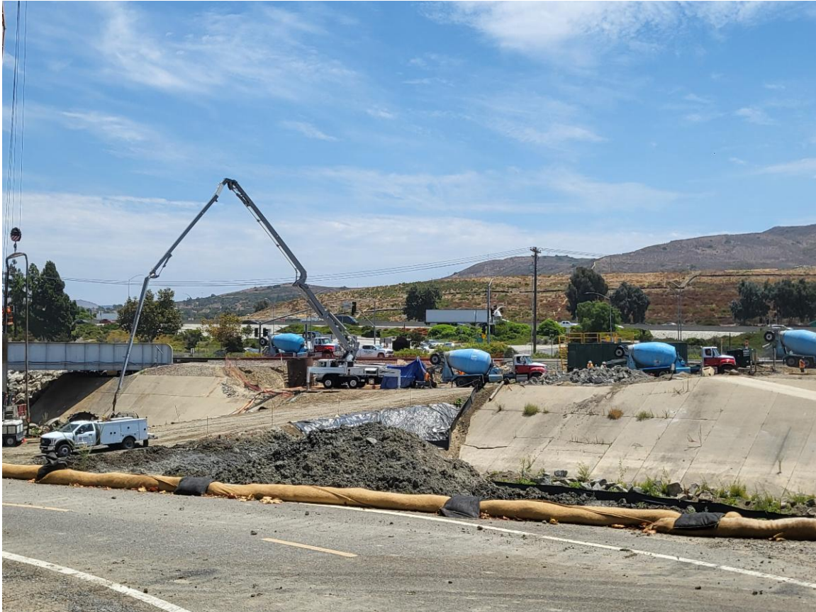
Concrete trucks staged next to the creek.
