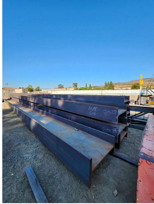
Piles that provide bridge support.
