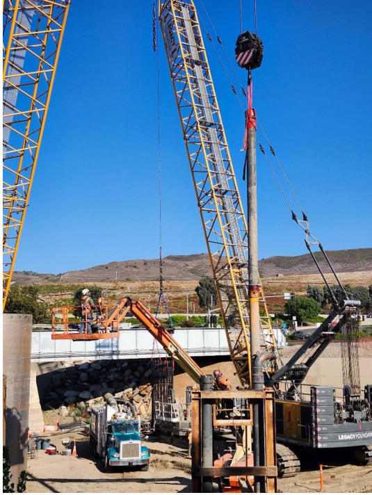
Crews installing bridge foundation.
