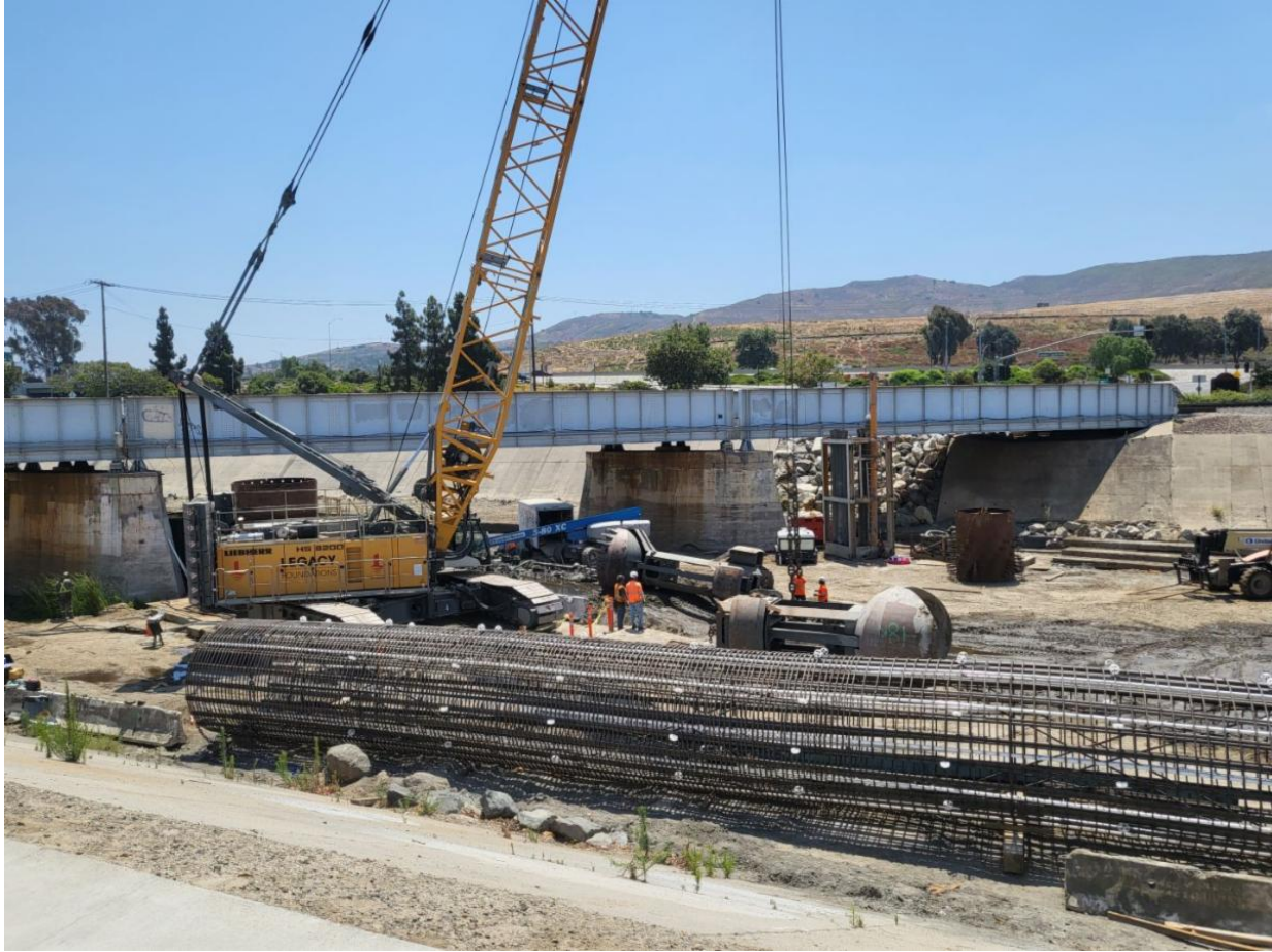
Crews working on bridge foundation in the creek
