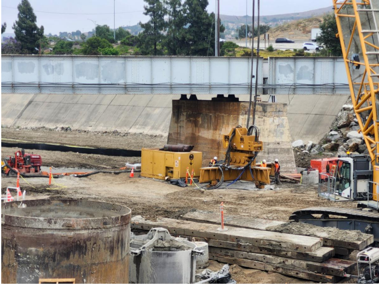
Bridge foundation work within San Juan Creek.
