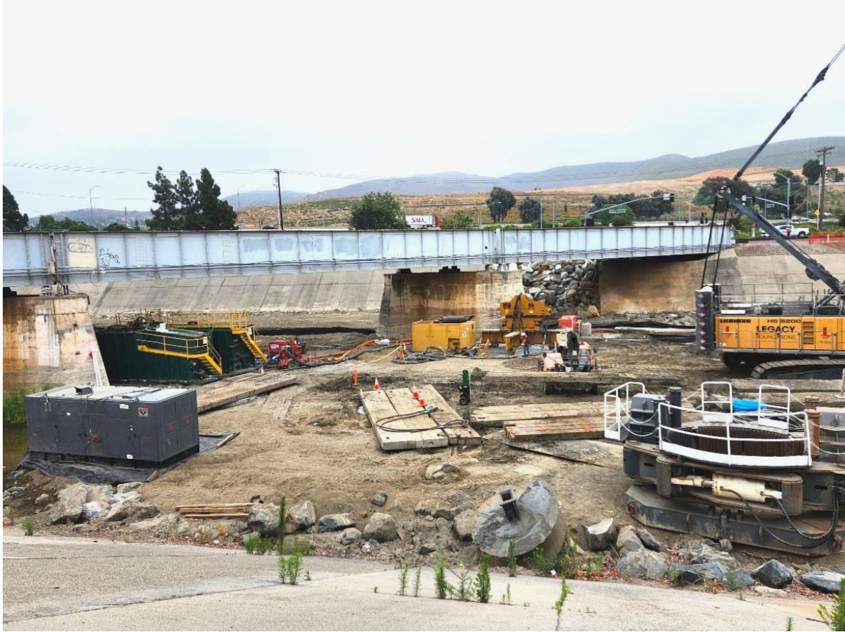
Bridge foundation work within San Juan Creek.
