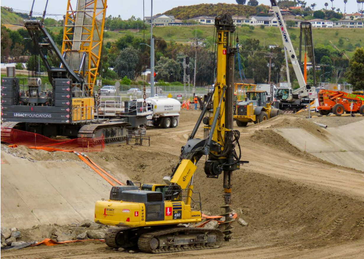
Drill rig mobilized to the project site.
