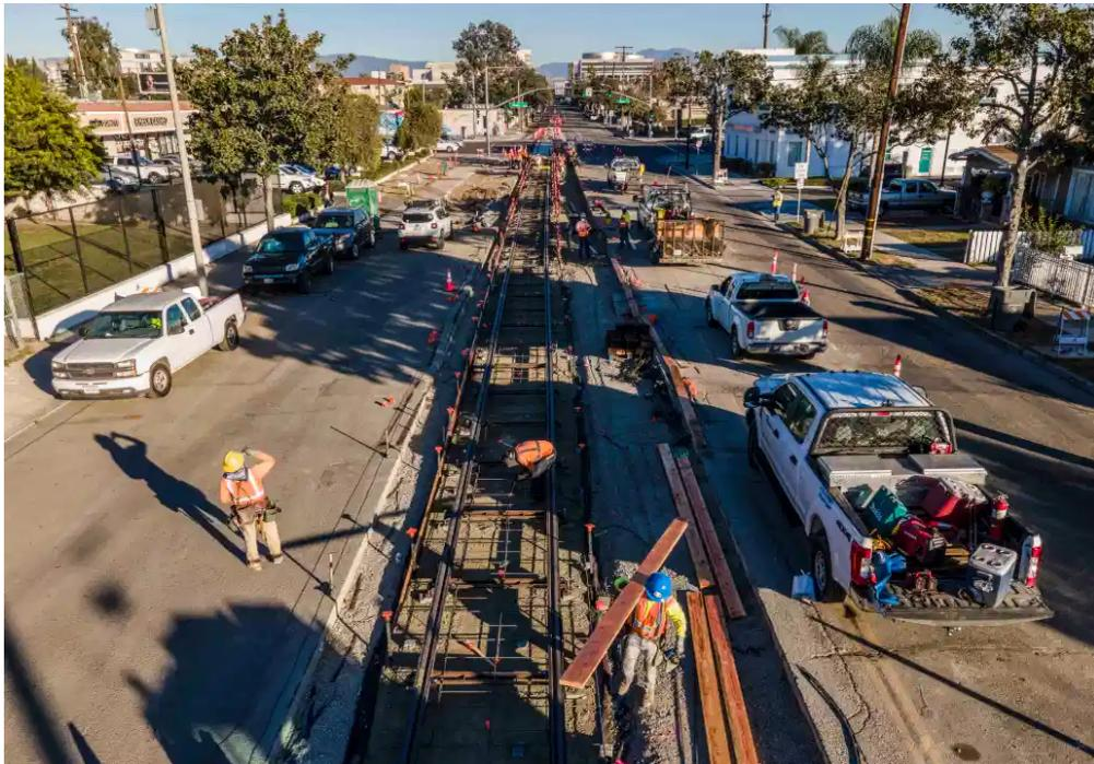
Rails are now being installed for OC Streetcar
