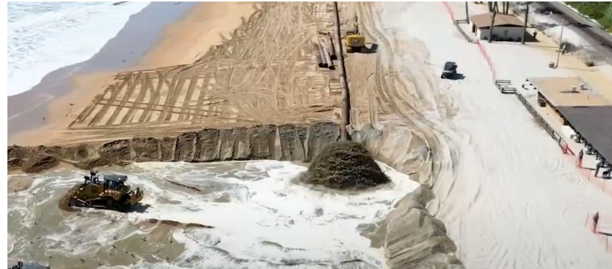
Pictures from San Clemente Sand Replenishment Project
