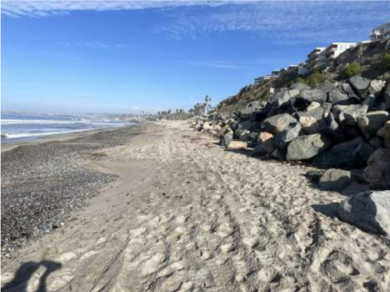
Figure 3 – Typical current site conditions at low tide from beach facing northwest, high beach berm in background
