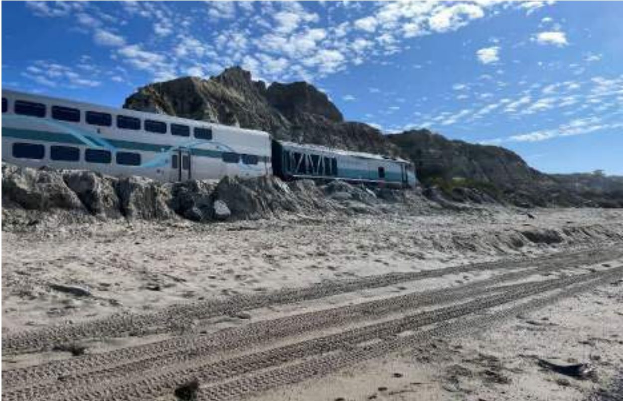
Figure 12 – Metrolink Train Passing Through Work Area in Proposed Northern Retention Repair
