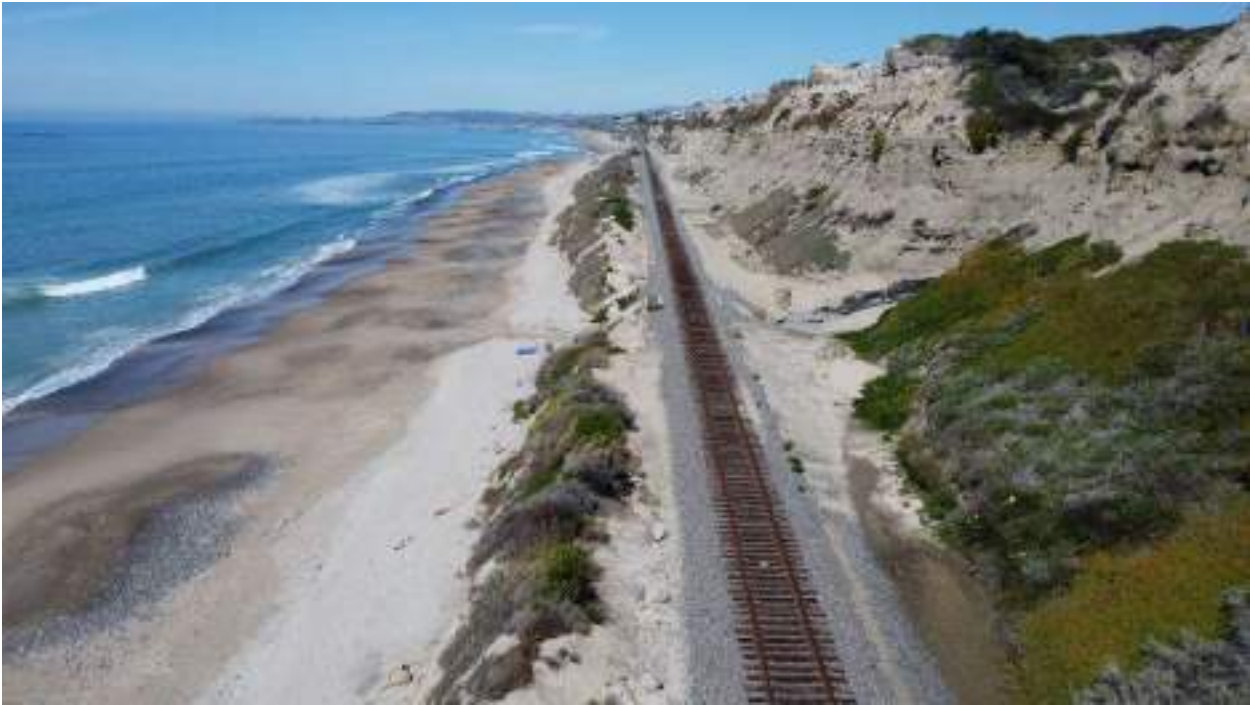
Figure 4 – Near Northern End of Proposed New Engineered Revetment, Replacing Eroded Berm And Vegetation
