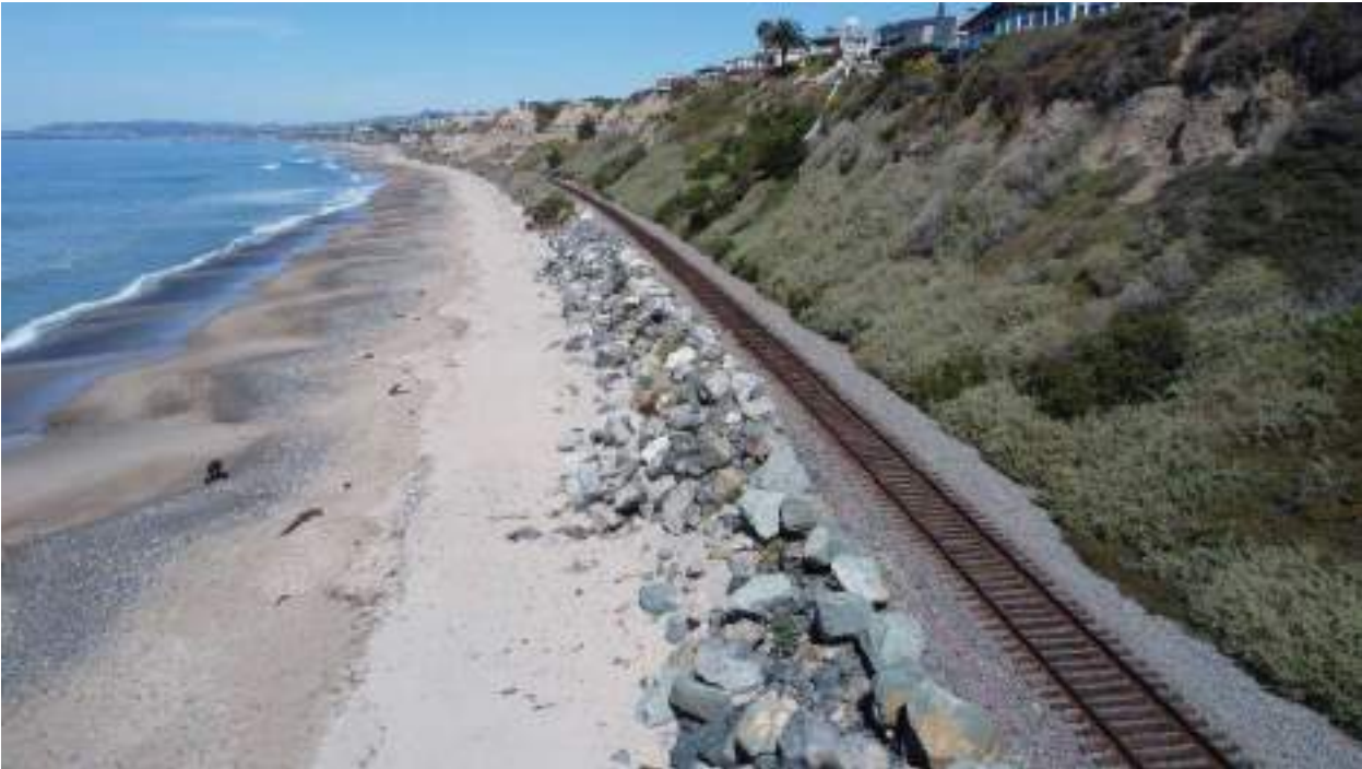
Figure 1 – Proposed Southern Riprap Area Near MP 206.7
