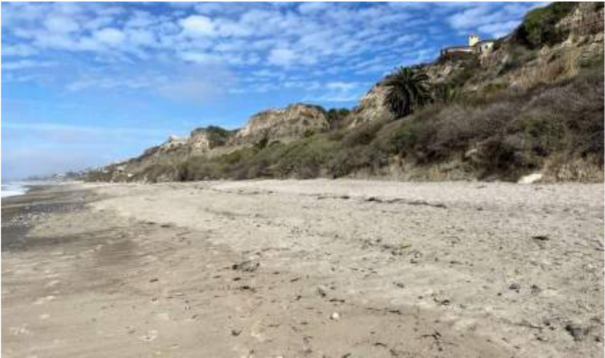
Figure 10 - Eroded berm in central portion of proposed new engineered revetment
