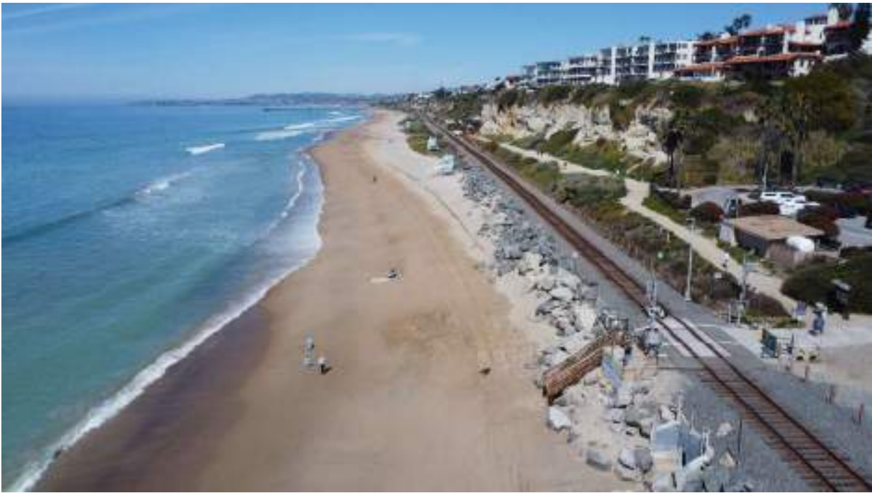
Figure 6 – End Of Proposed North Riprap Repair Near Pedestrian Crossing, Stairs and Culvert at MP 206.00
