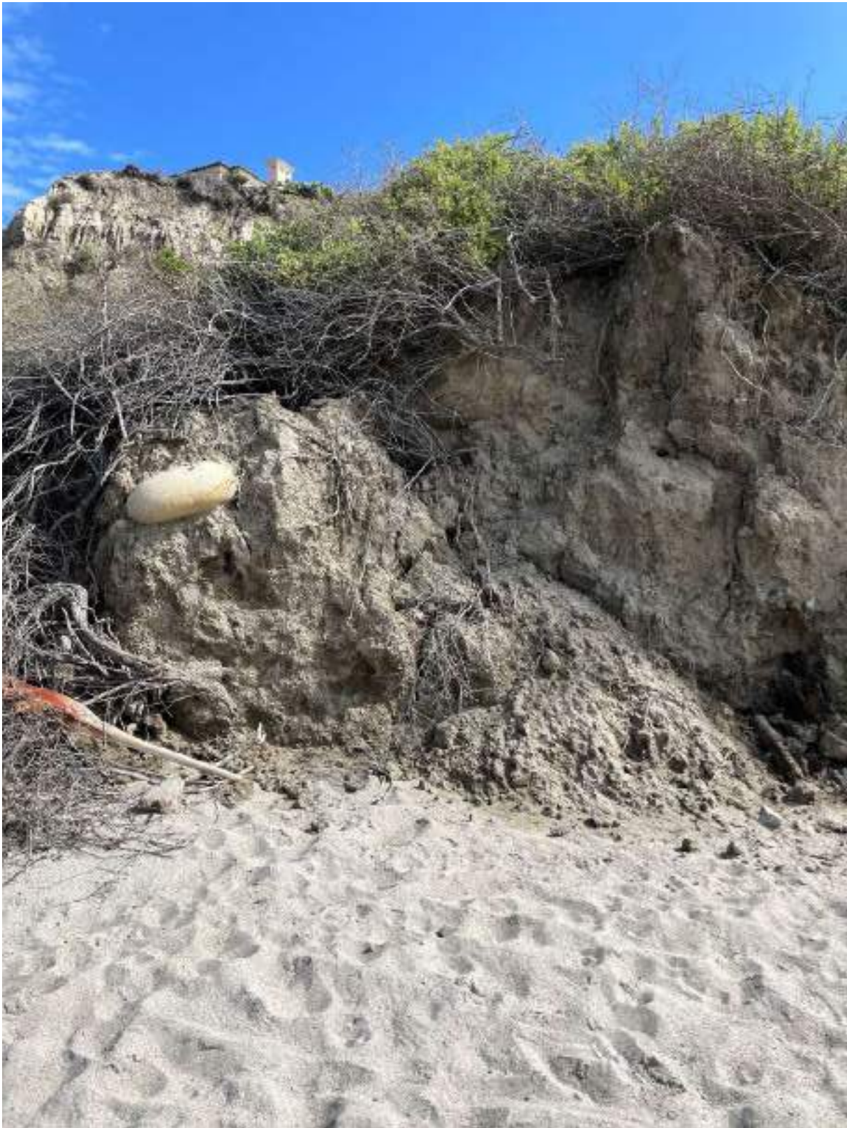
Figure 11 - Eroded Berm at North End of the Proposed Engineered Revetment
