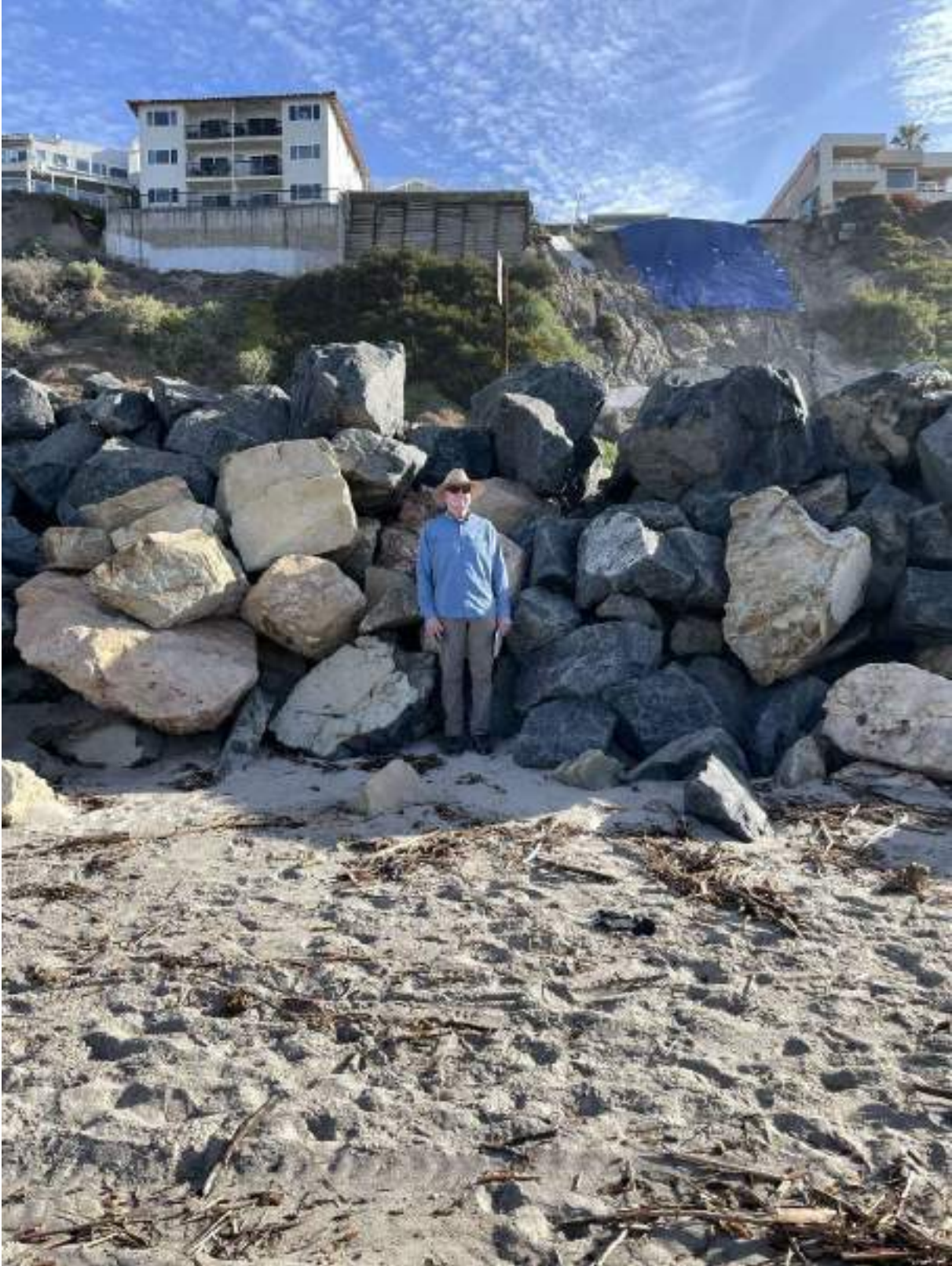
Figure 2 – Typical current site conditions from lower beach, over-steepened riprap central image
