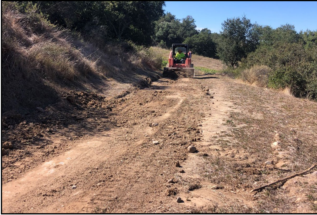
PHOTOGRAPH 29 Recontouring of Fire Road to Repair Erosion Rills, Live Oak Creek Preserve, November 2023
