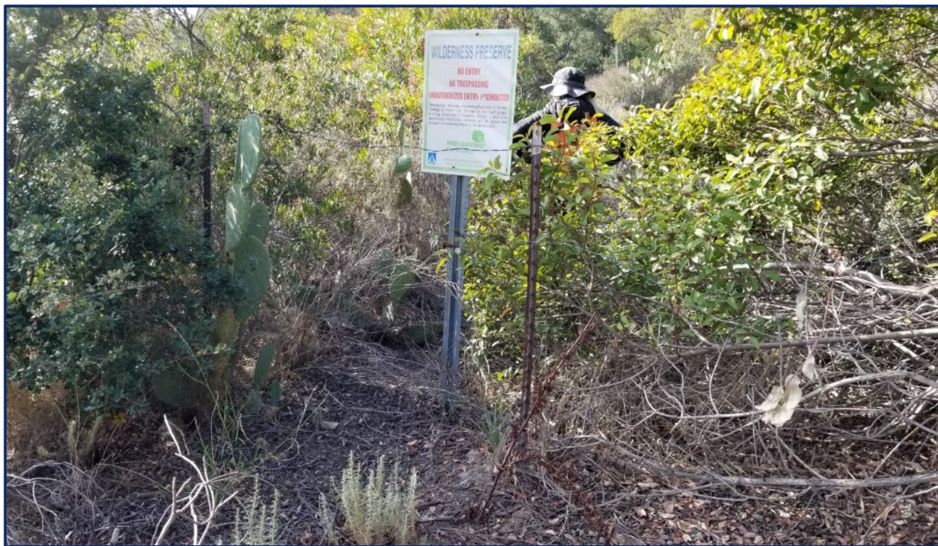
Photograph 11: Depicting area in need of fence repair. Photo taken December 7, 2023.
