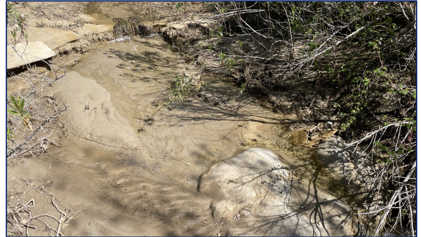
Photograph 18: Southwestern pond turtle pond shown filled in with sediment. Photo taken March 7, 2023.
