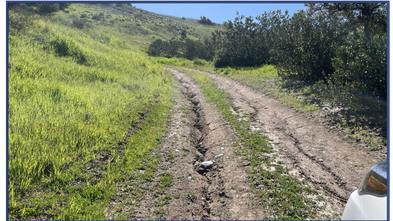
Photograph 4: Depicting erosion along main access road. Photo taken February 20, 2023.
