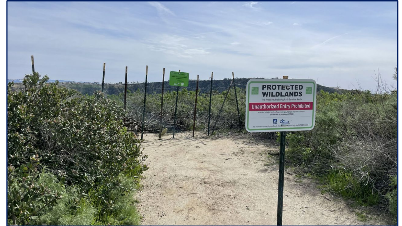
Photograph 2: Depicting repaired fence and newly installed signage to deter trespassers. Photo taken February 17, 2023.
