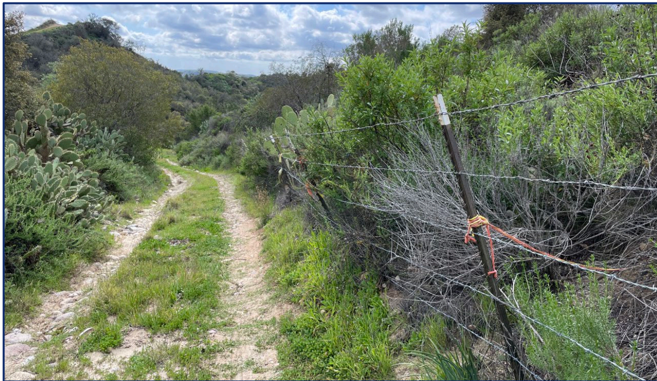
Photograph 3: Depicting barbed wire fence leaning into roadway. This fencing has now been removed. Photo taken February 13, 2023.
