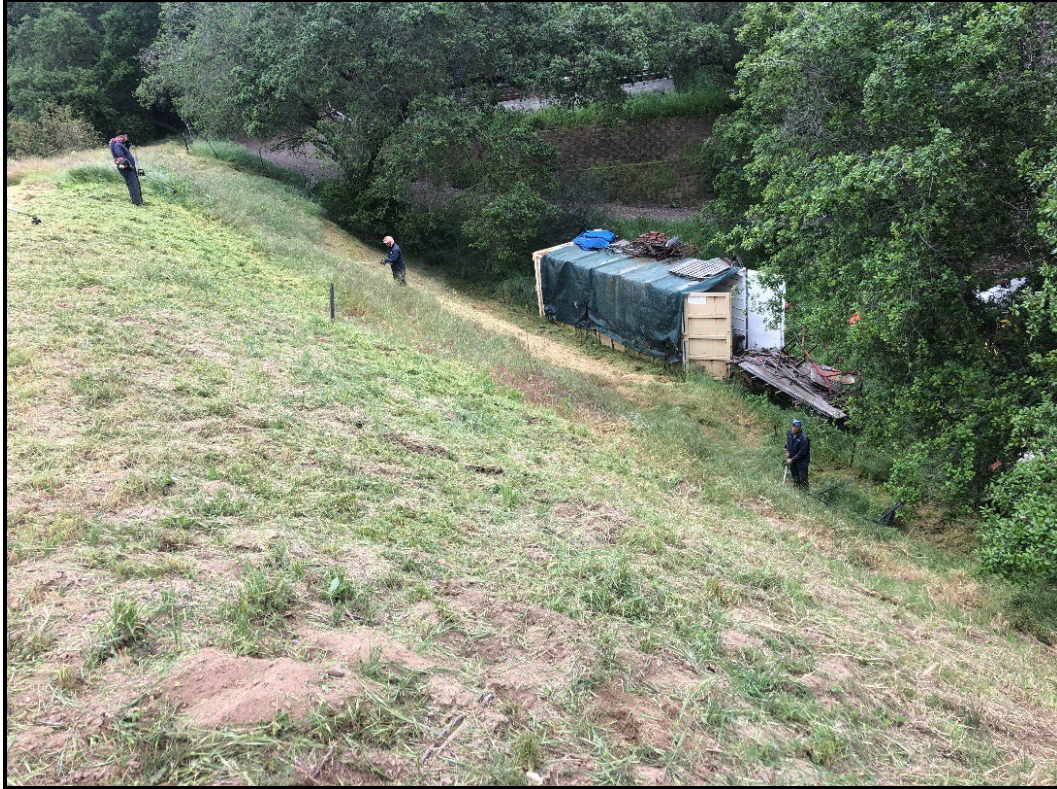
PHOTOGRAPH 5 Fuel Modification Work Near 20022 Trabuco Oaks Drive, Trabuco Rose Preserve, April 2023
