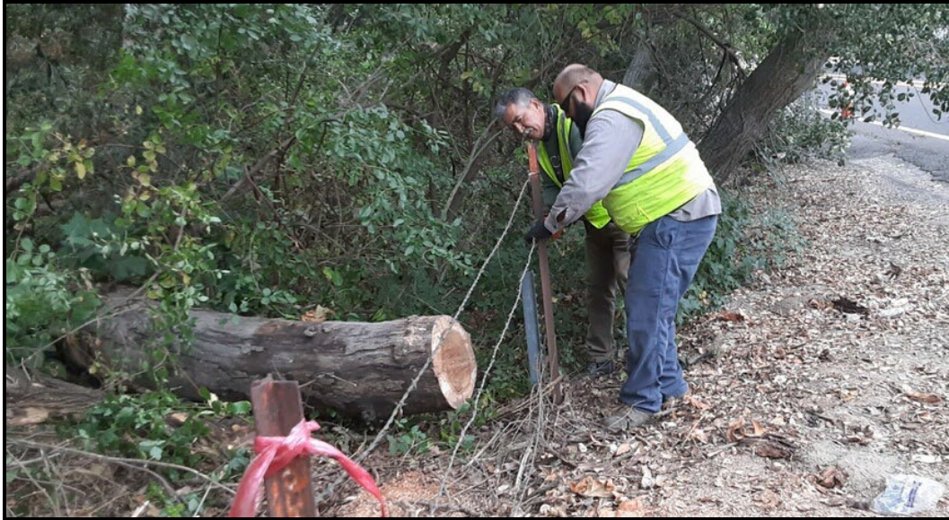
PHOTOGRAPH 26 Repairs Made to Damaged Fence Line, Live Oak Creek Preserve, August 2023
