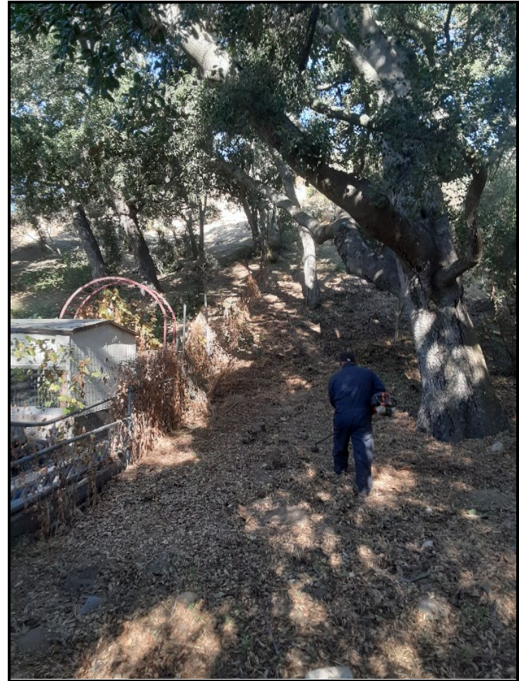
PHOTOGRAPH 10 Fuel Modification Work Near 2021 Trabuco Oaks Drive, Trabuco Rose Preserve, July 2023
