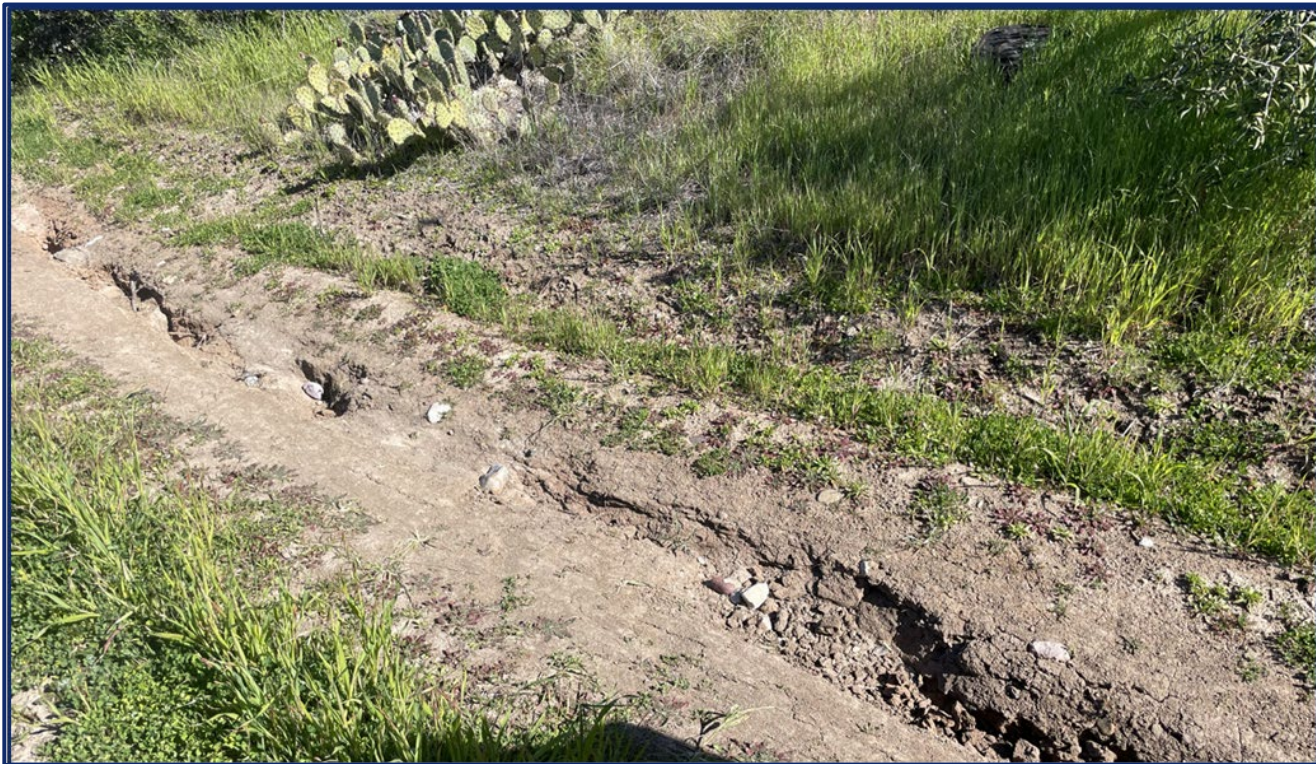
Photograph 3: Depicting deep erosion along main access road. Photo taken February 20, 2023.
