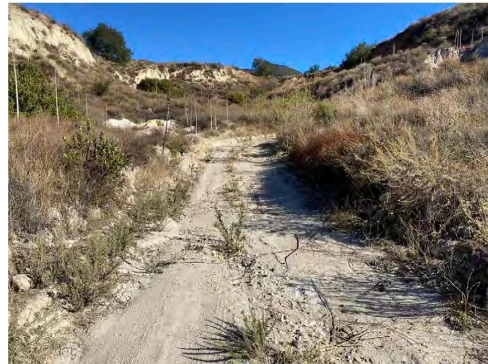
Photograph 12: View of road in need of maintenance – vegetation removal and filling in erosional areas. Photo taken December 22, 2020.
