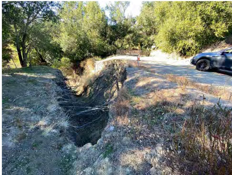
Photograph 11: View of large area of stream erosion adjacent to the access road east of the main gate (near the secondary gate). Photo taken December 22, 2020.
