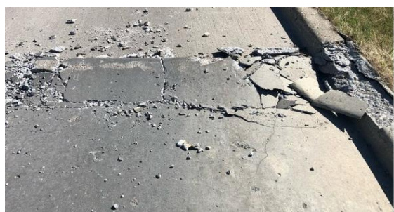
Figure 4-3. Road Buckling 26
