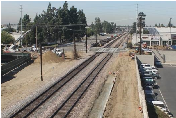
Photo: Time lapse camera facing east at State College Boulevard
