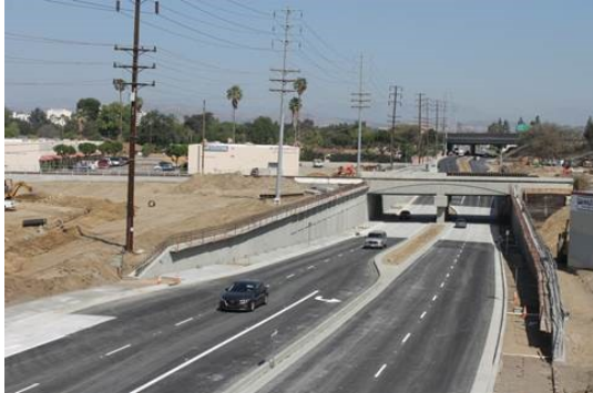
Photo: Looking north at new Placentia Avenue bridge
