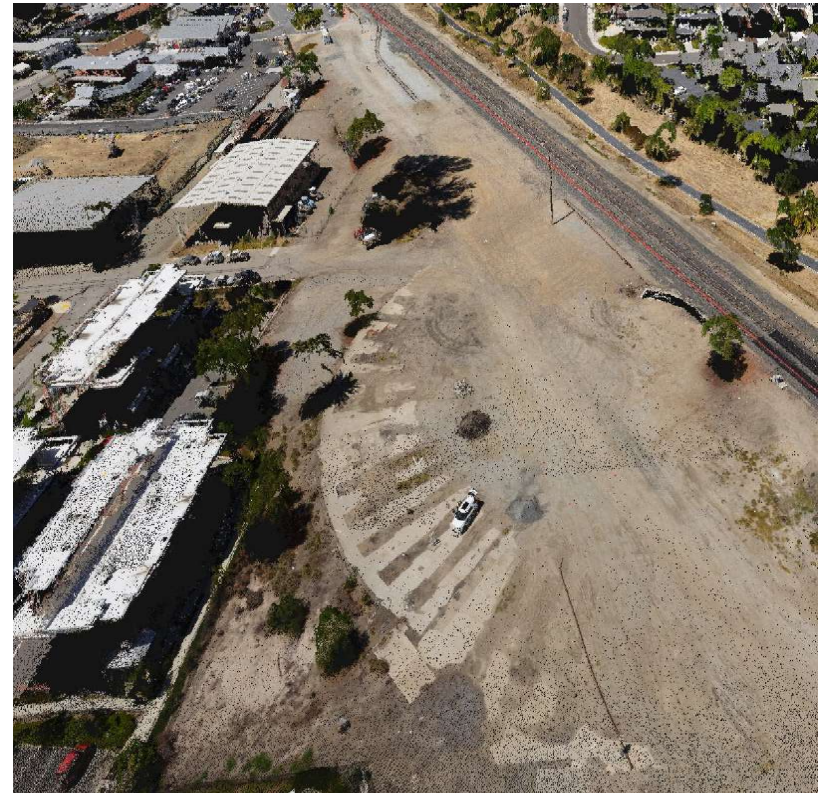
Figure 10-9 of Draft EIR Appendix E. Oblique Aerial Image of the Roundhouse Foundations as They Appeared in October 2020, Facing North
