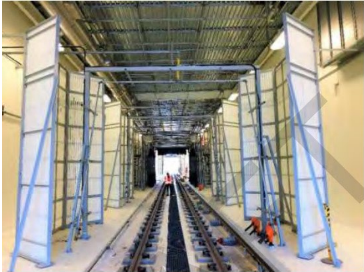
Figure 2-3. Typical Automatic Drive-Through Train Wash
