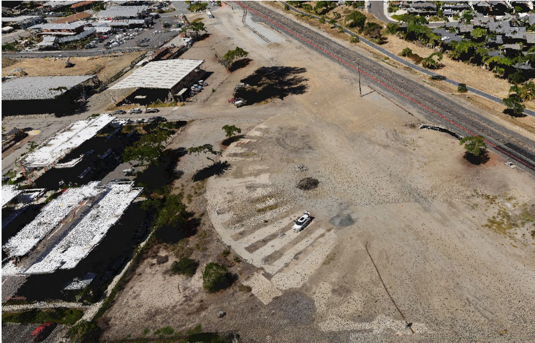
Figure 3.5-4. Oblique Aerial Image of the Roundhouse Foundations as They Appeared in October 2021, Facing North
