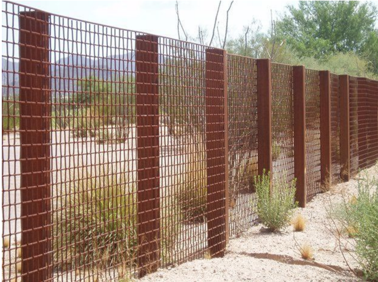
Figure 3.2-12. Welded Wire Mesh Fencing Example
