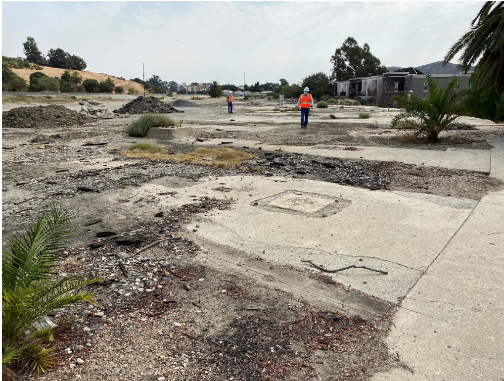
Figure 3.5-5. Overview of Roundhouse Foundations Facing South-Southeast
