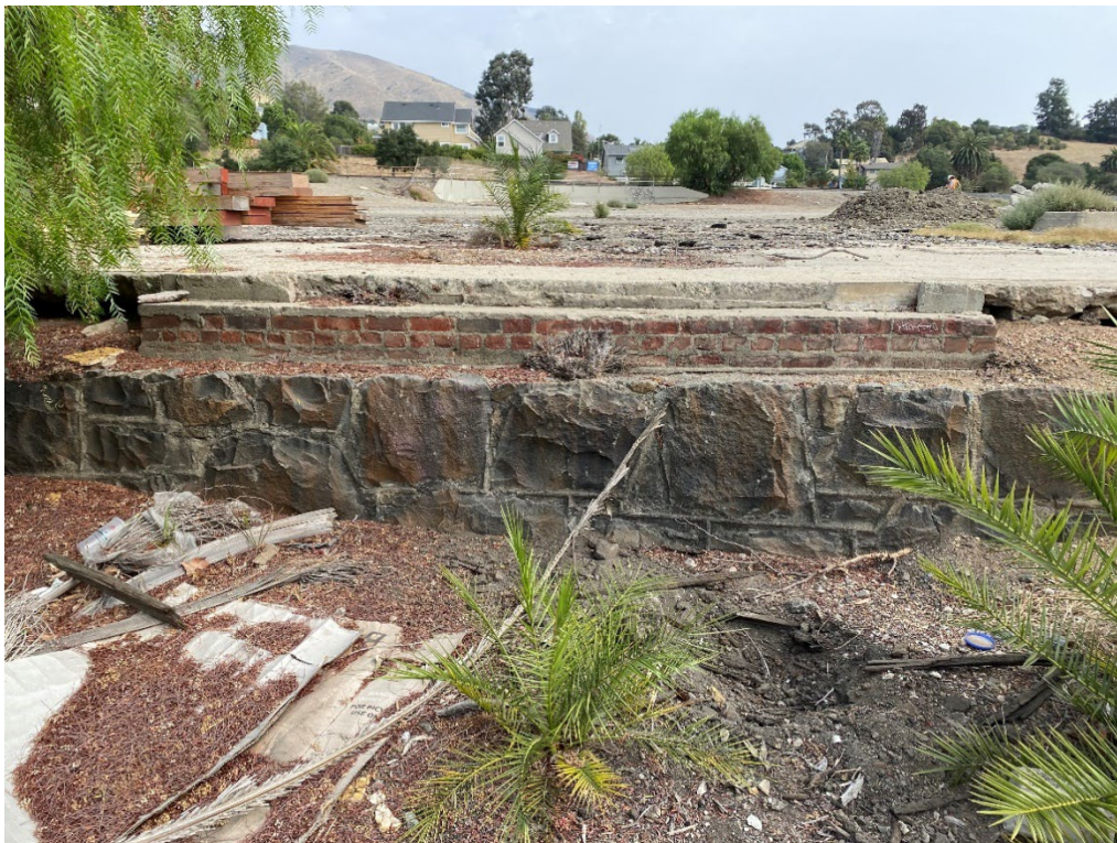
Figure 3.5-6. West Profile of Roundhouse Showing Cut-Stone Retaining Wall and Brick Section, Facing East
