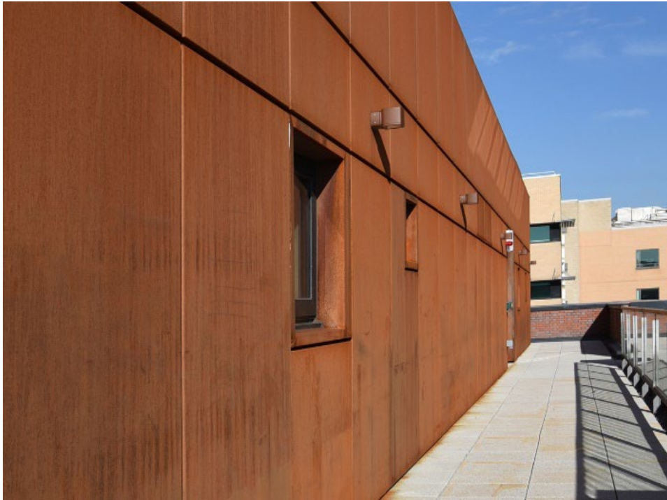
Figure 3.2-10. Corten/Weathering Steel Rainscreen
