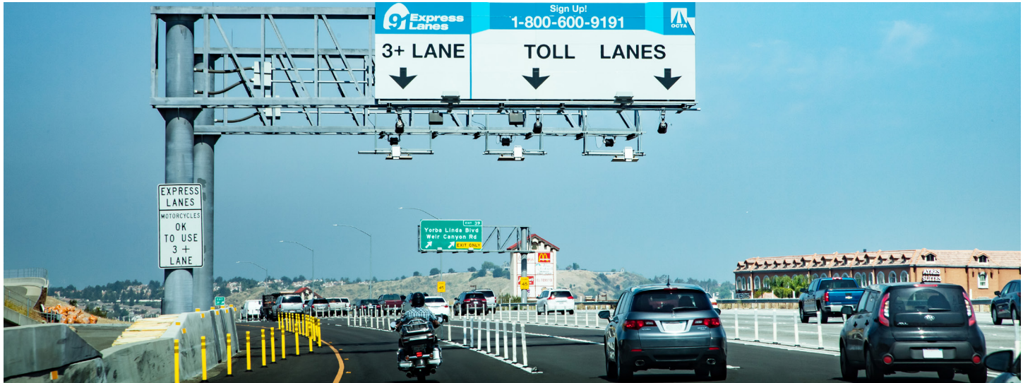
91 Express Lanes toll gantry and signage.
