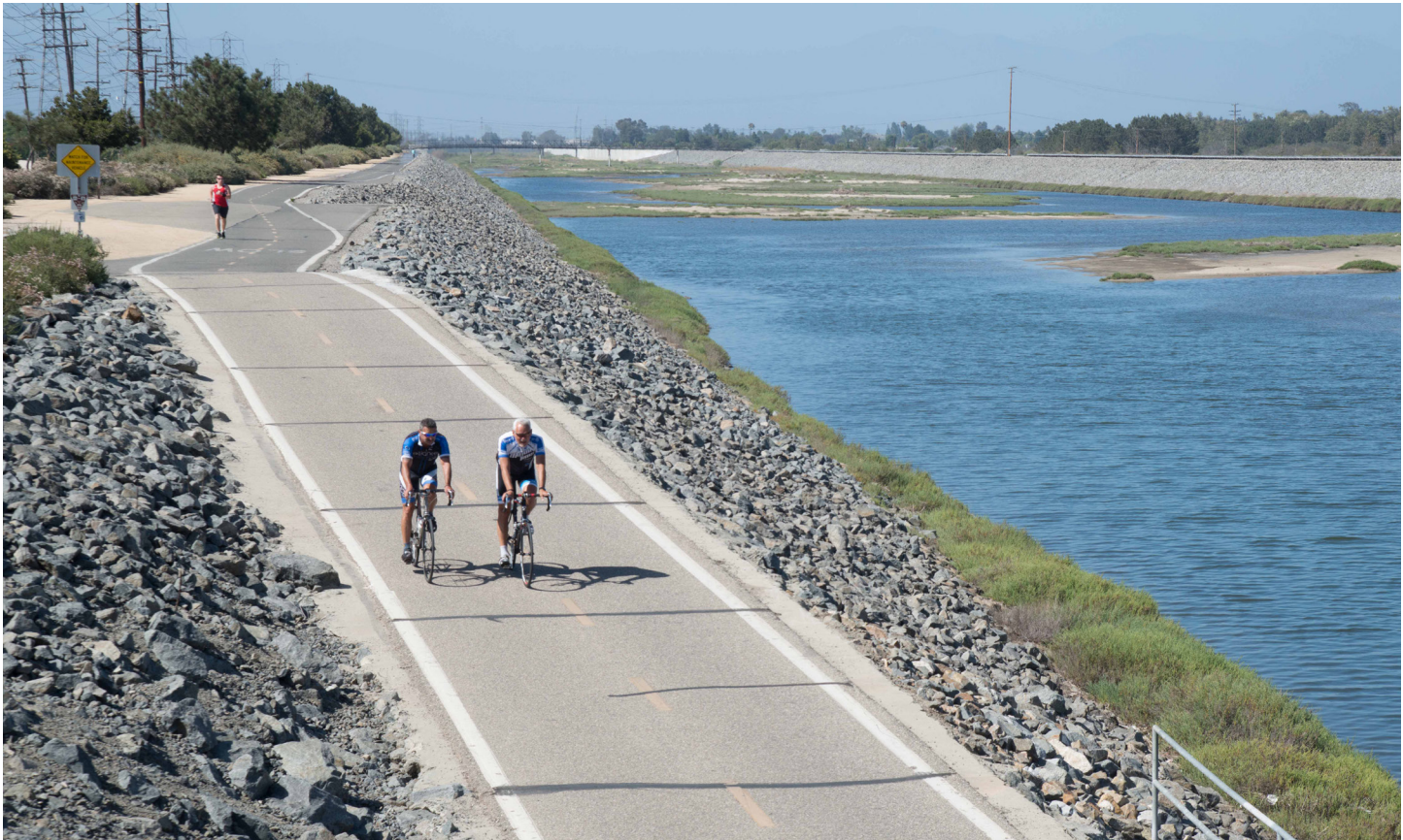
Bicycle and pedestrian facilities promote active transportation.
