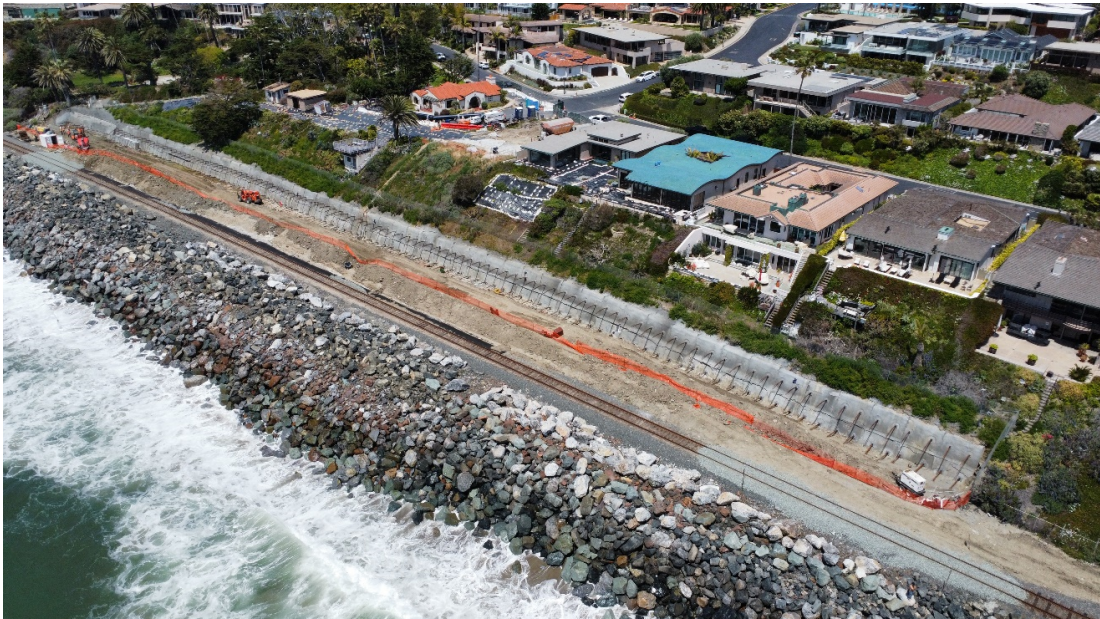
Figure 1 MP 206.8 Track Stabilization Project (Cyprus Shore)
