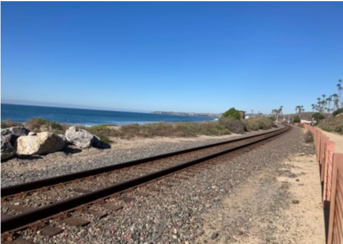
Figure 8. Monitoring Site 3: MP 203.65, North Beach
