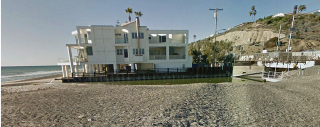
Figure 7. Monitoring Site 2: MP 202.70, Poche Beach Outfall and Pedestrian Underpass
