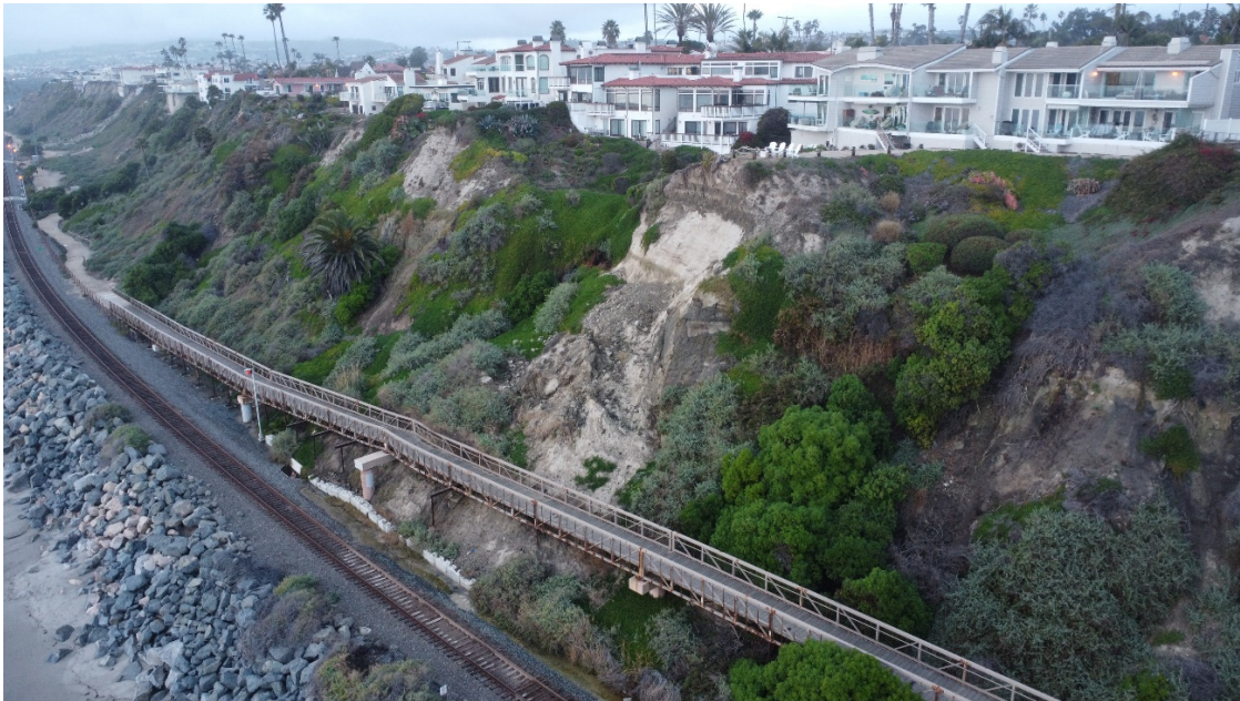
Figure 9. Monitoring Sites 4 and 5: MP 204.1–204.3, Mariposa Pedestrian Bridge – January 21, 2024.
