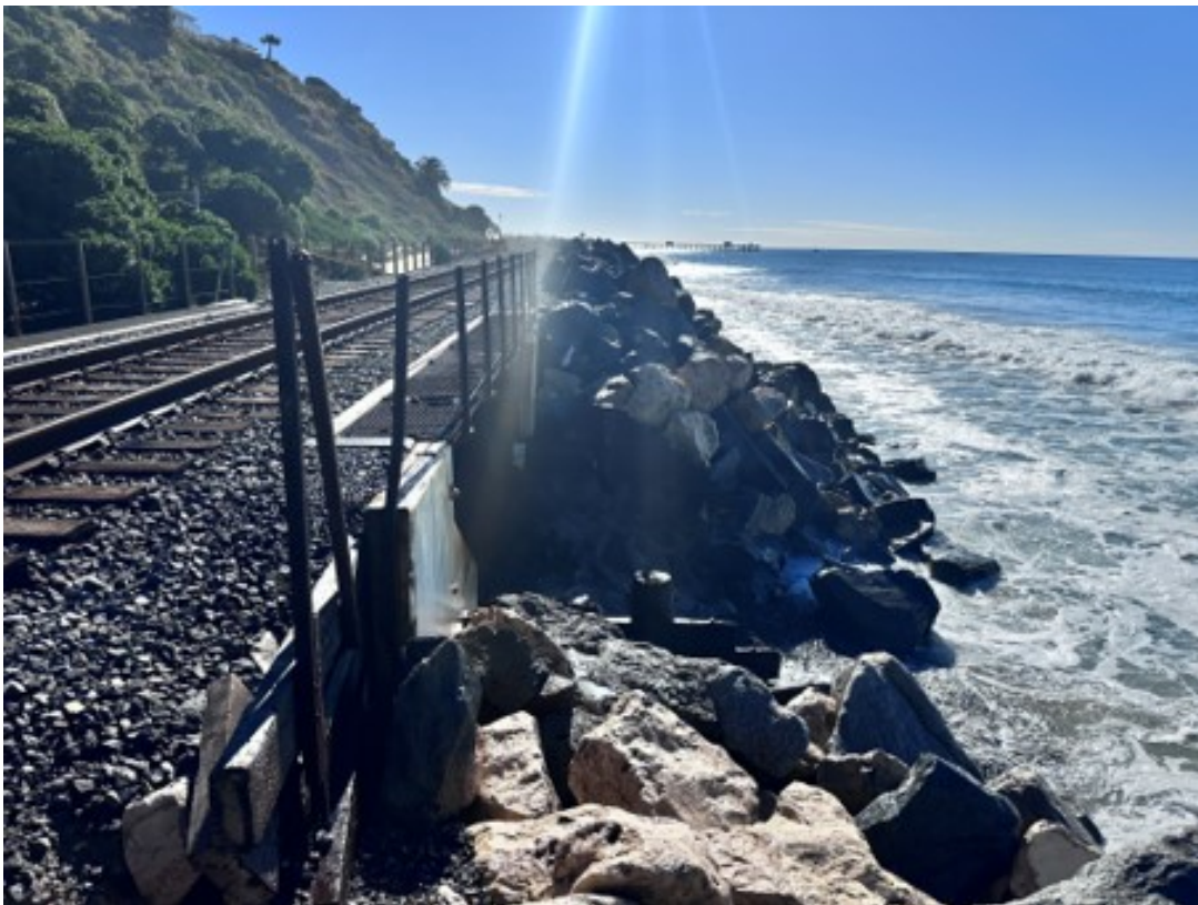
Figure 14. Potential Reinforcement Site 2: MP 204.00 to MP 204.40
