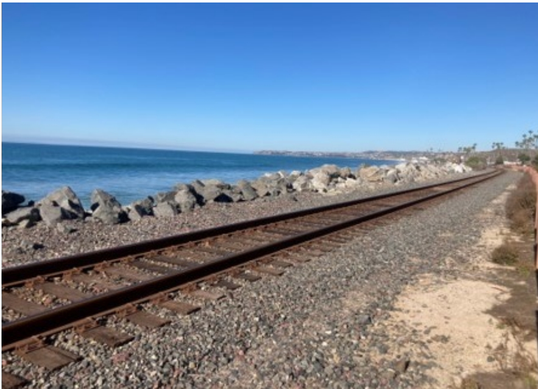
Figure 12. Potential Reinforcement Area 1: MP 203.85 to MP 203.90
