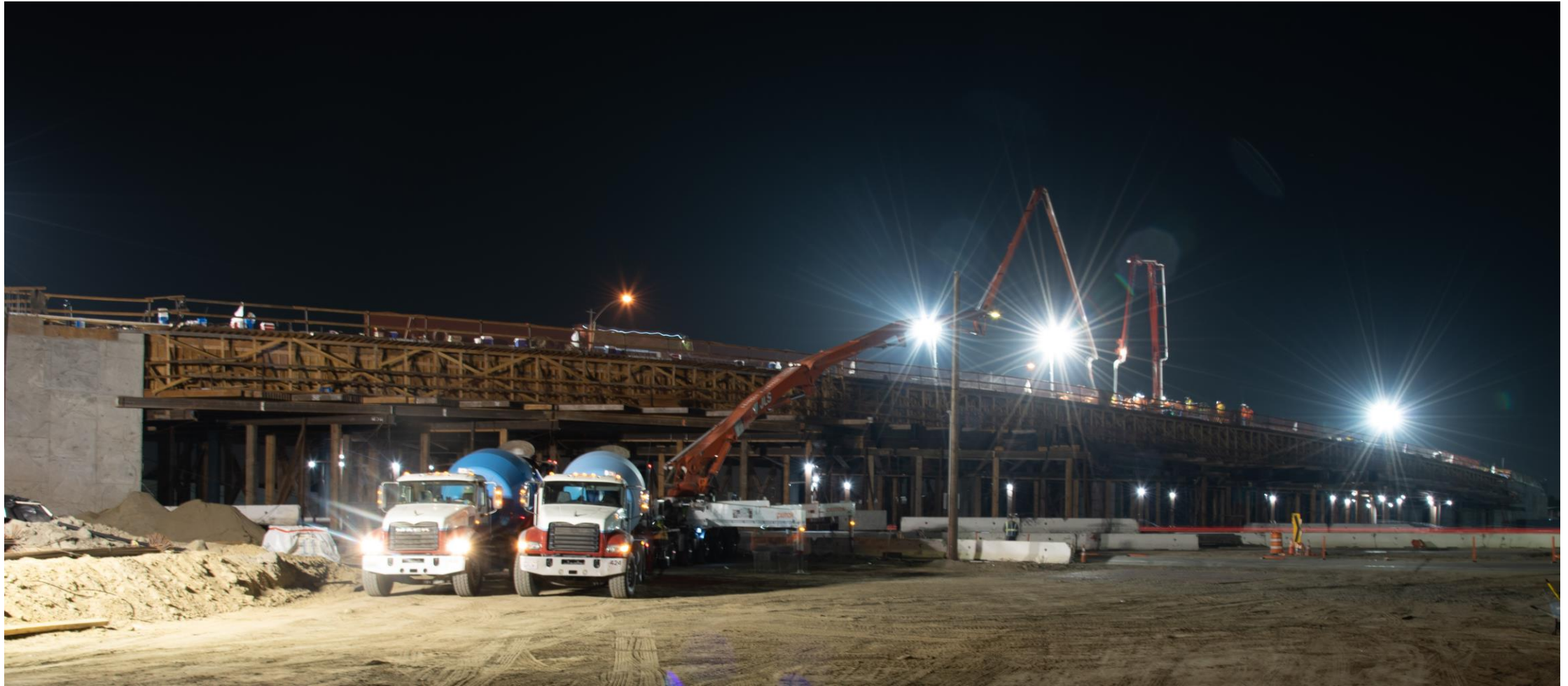
Bolsa Avenue bridge construction
