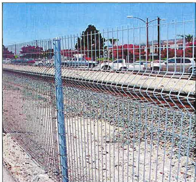
Figure 10-3: Example of a “No-Climb”-type fence used by Metrolink along its rail right-of-way
