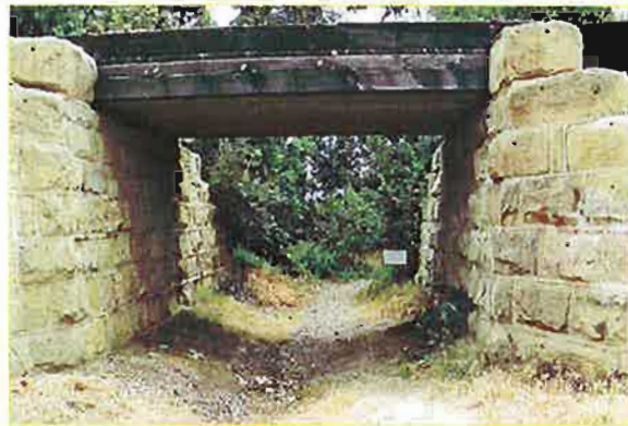
Figure 4-21: Existing drainage crossing east of Calle Ocho
