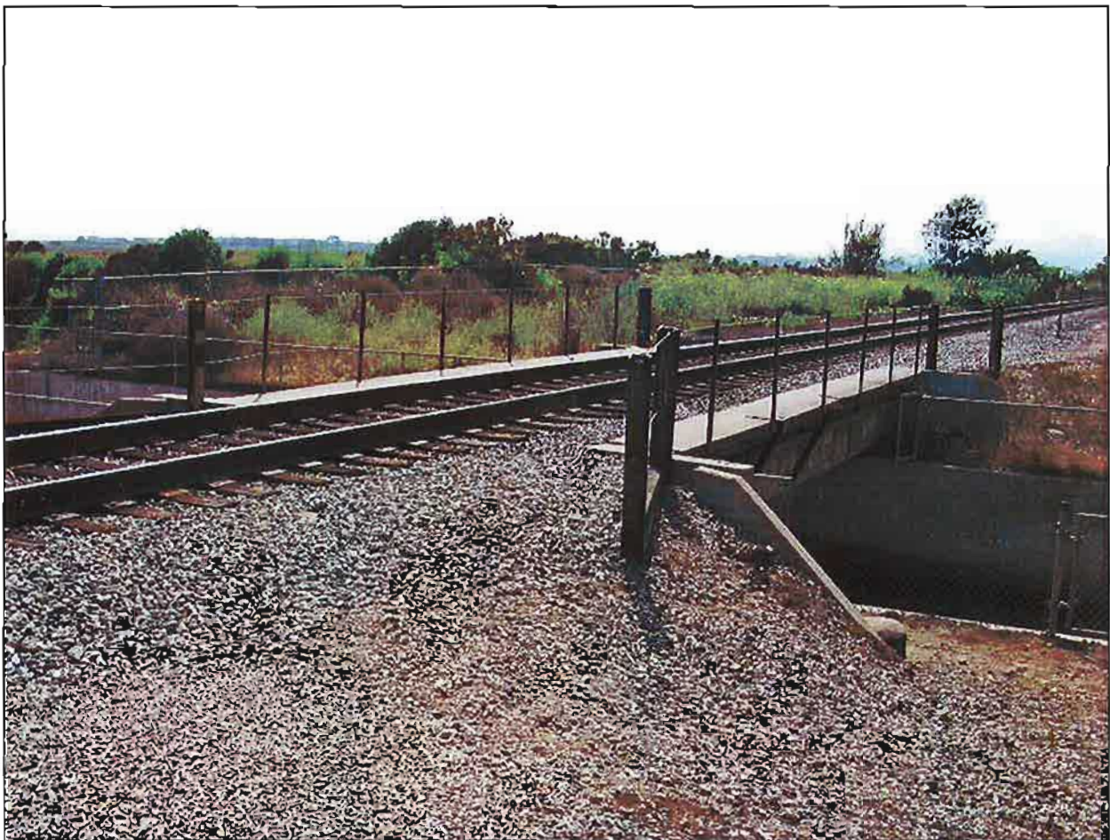
Figure 4-40: Railroad bridge over Franklin Creek, looking west
