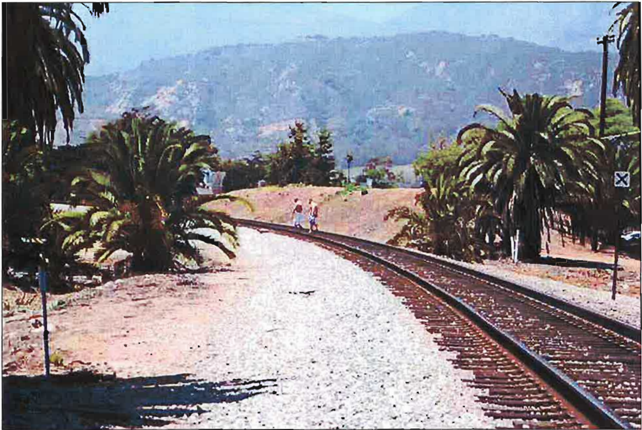
Figure 4-36: View from the rail ROW near Holly Avenue, looking west
