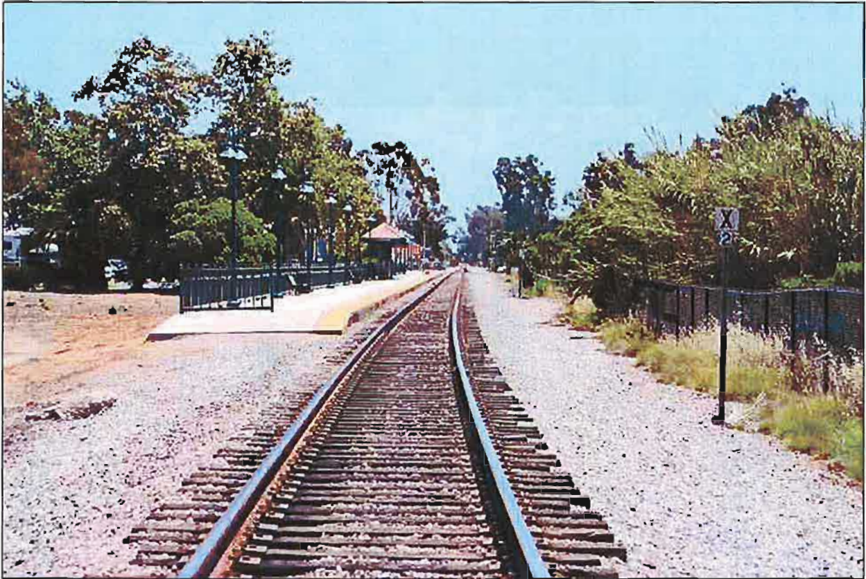
Figure 4-35: Rail ROW from near Holly Avenue, looking east
