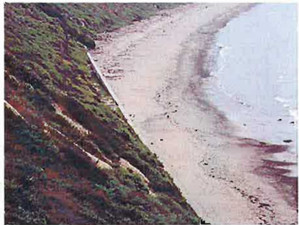
Figure 4-7: Steep drop-off between rail corridor and bluffs limits easy access to the coastline between Carpinteria and Rincon County Beach
