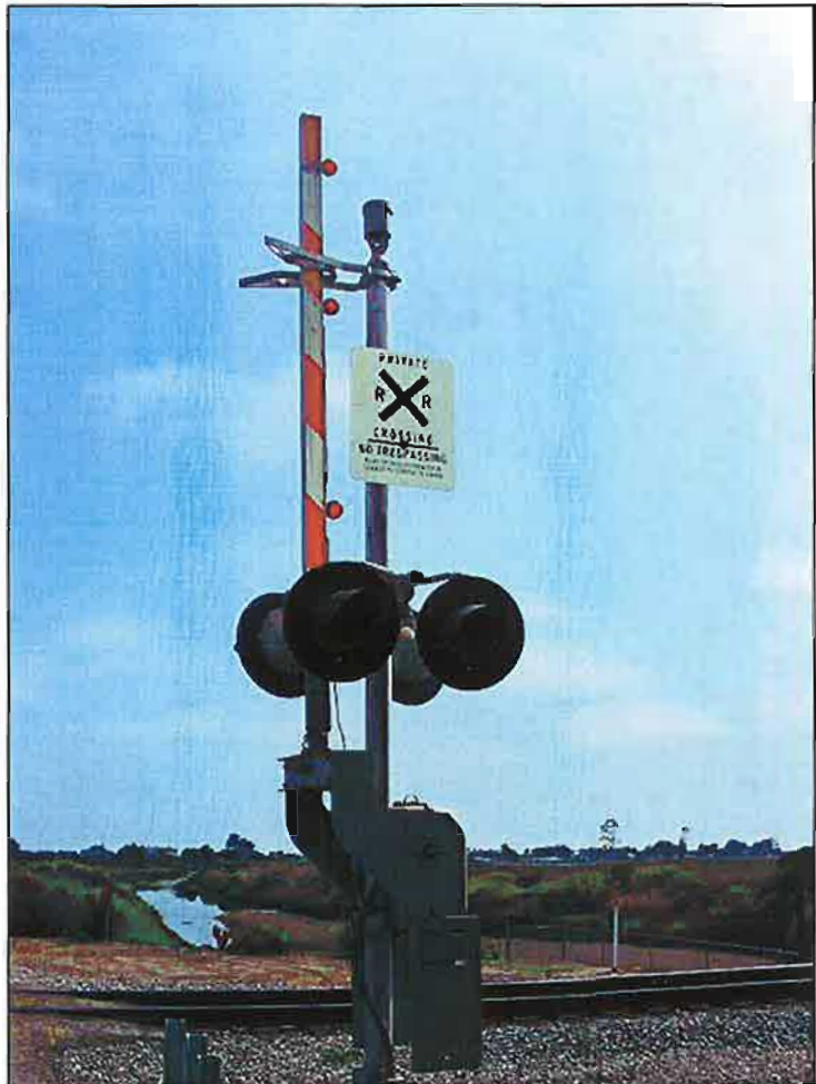
Figure 4-43: Private railroad crossing at Sandyland Cove Road
