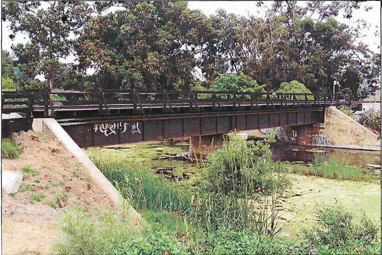
Figure 4-27: Rail structure over Carpinteria Creek, looking southeast
