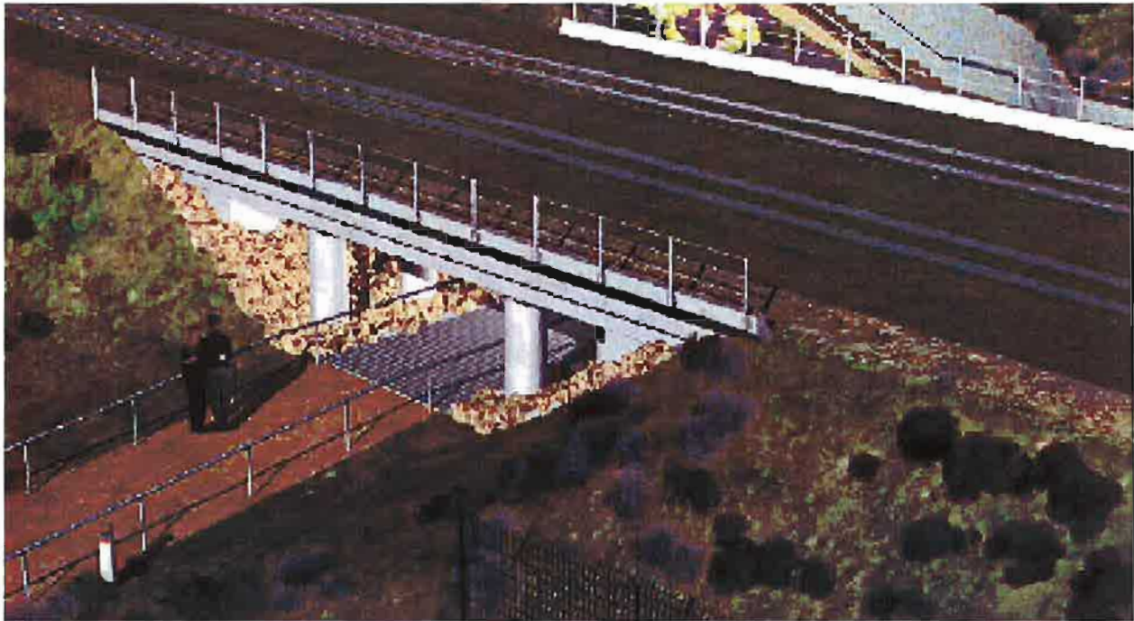
Figure 9-1: Artist's rendering of a conceptual UPRR Standard Precast Concrete Box Girder Underpass (Source: City of Encinitas)
