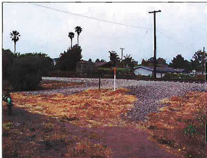
Figure 8-2: Potential Calle Ocho access crossing location as viewed from Tar Pits Park, looking north
