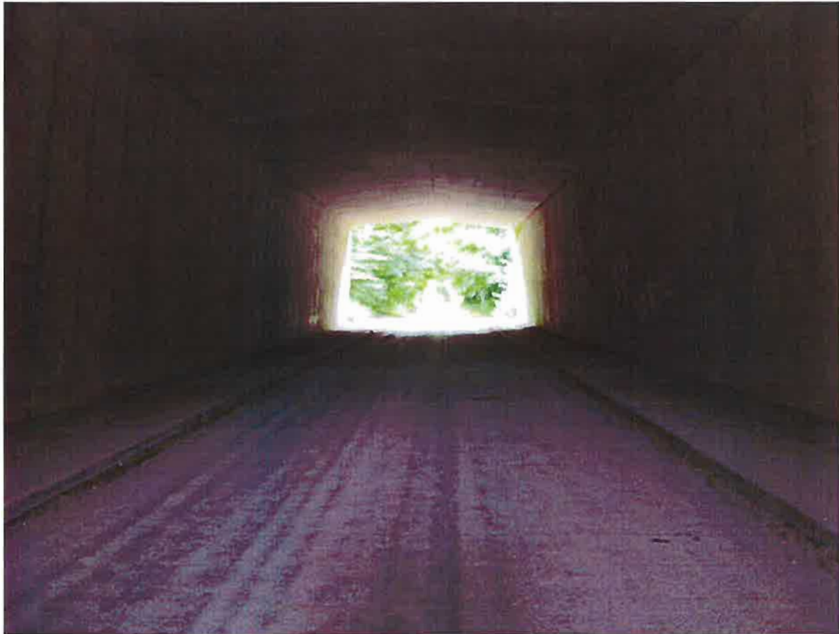
Figure 9-4: Example of Concrete Box Tunnel (Typical) (Photo Credit/Copyright: Dr. Duncan Pepper 13 )
