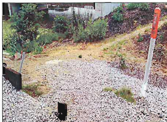
Figure 4-28: Evidence of unsanctioned access between rail bridge and pedestrian bridge near Carpinteria Creek
