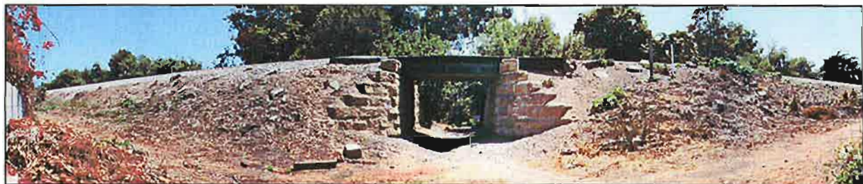
Figure 4-22: Panoramic view of existing drainage under crossing near Calle Ocho
