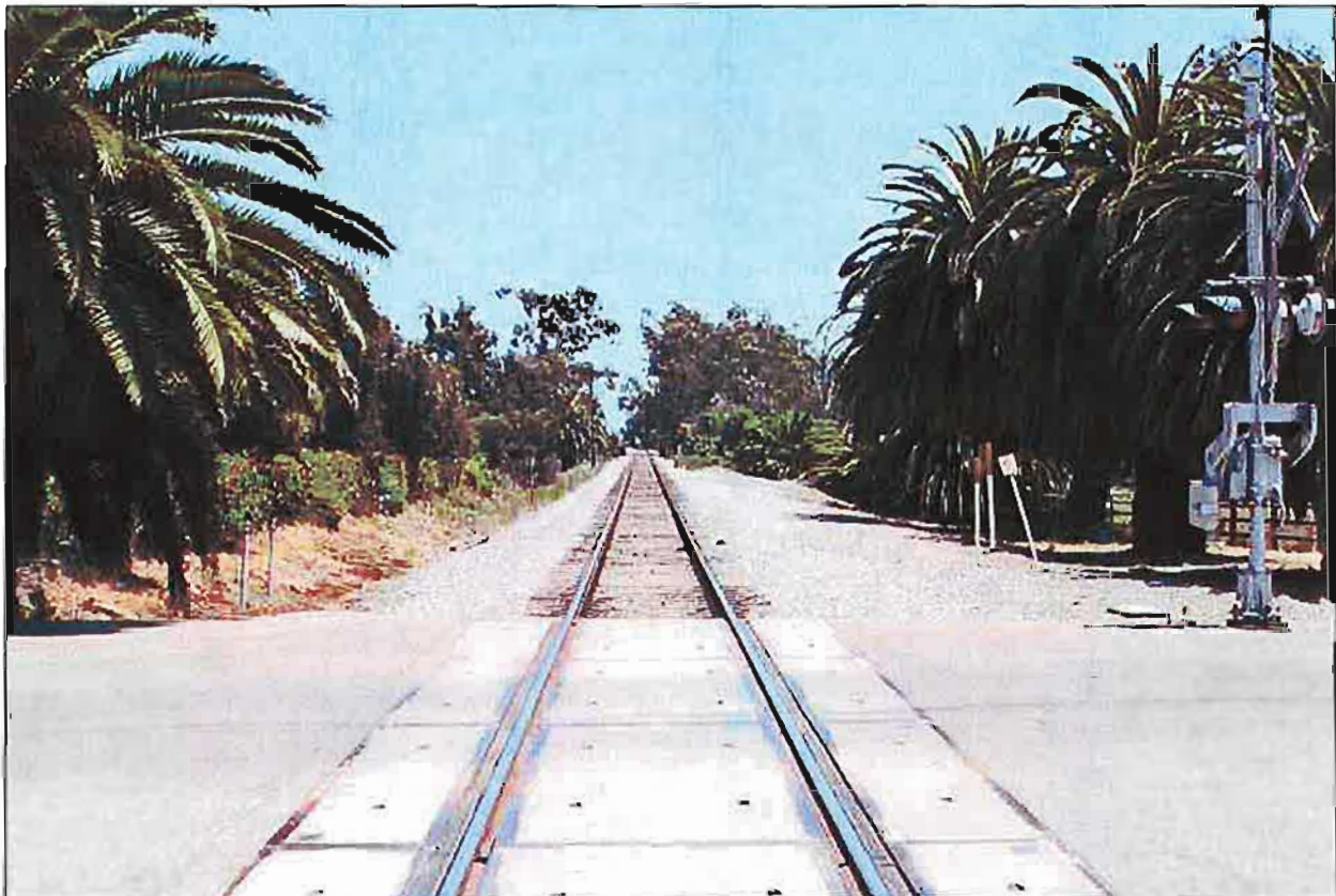
Figure 3-1: Palm Avenue Crossing, looking east toward Carpinteria Creek – one of only two sanctioned public at-grade crossings in the City
