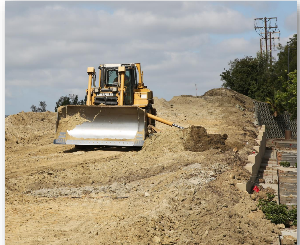
Bulldozer working near La Paz Road.
