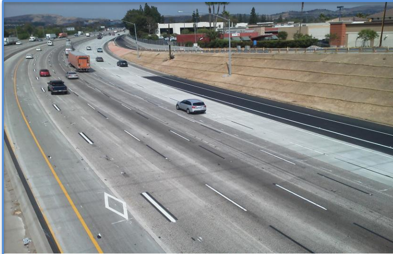
5-mile northbound general purpose lane addition
