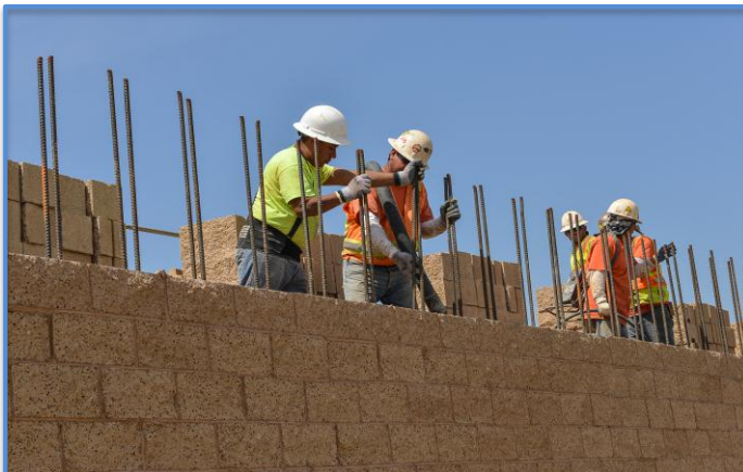
More than 3 miles of sound walls
