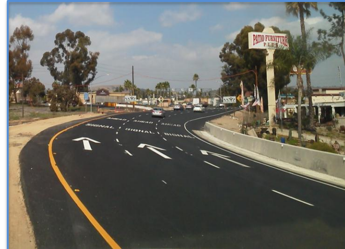
12 ramps realigned and reconstructed
