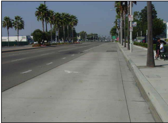
Photo 8: Concrete pad at bus stop.
