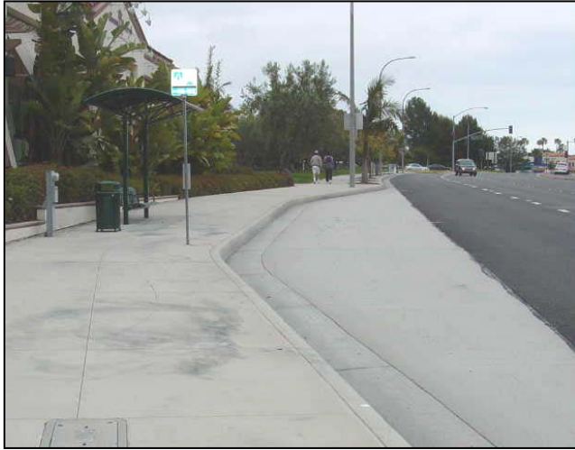
Photo 7: Typical “mid-block” type turnout on arterial street.
