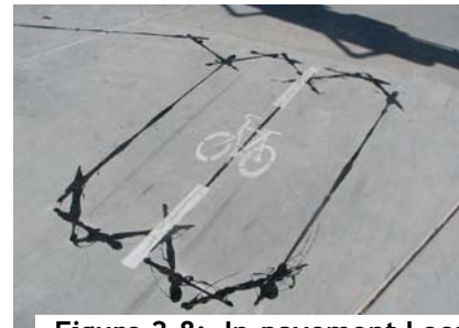
Figure 2.8: In-pavement Loop Detector
