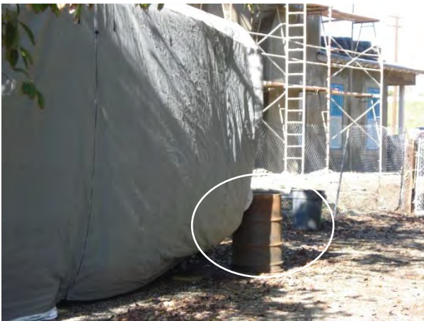
Photo 3A – Residential Property (29931 Camino Capistrano, San Juan Capistrano). This site is to a residential property. An unlabeled 55-gallon metal rusted drum was noted.
