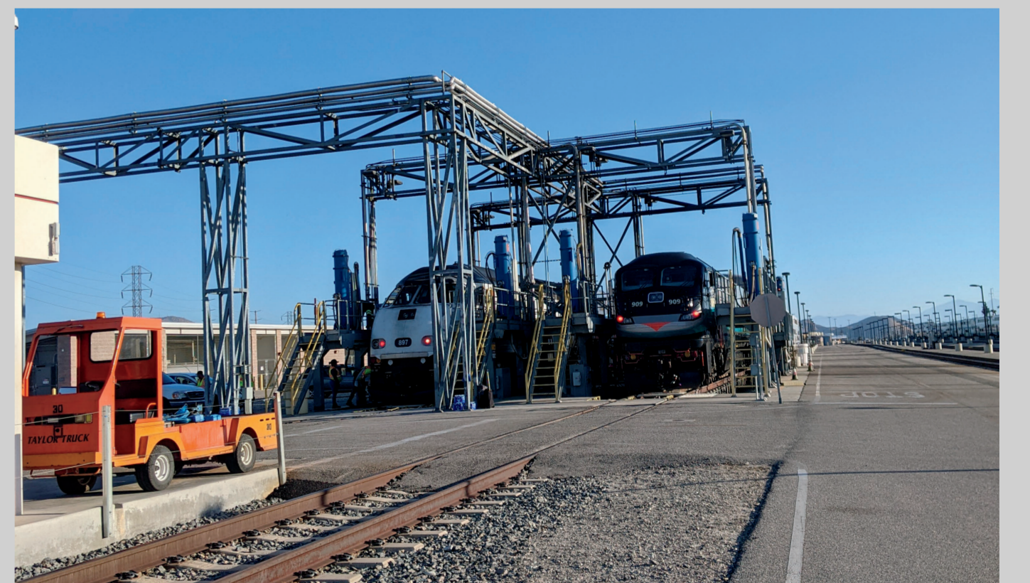
Service & Inspection Station
