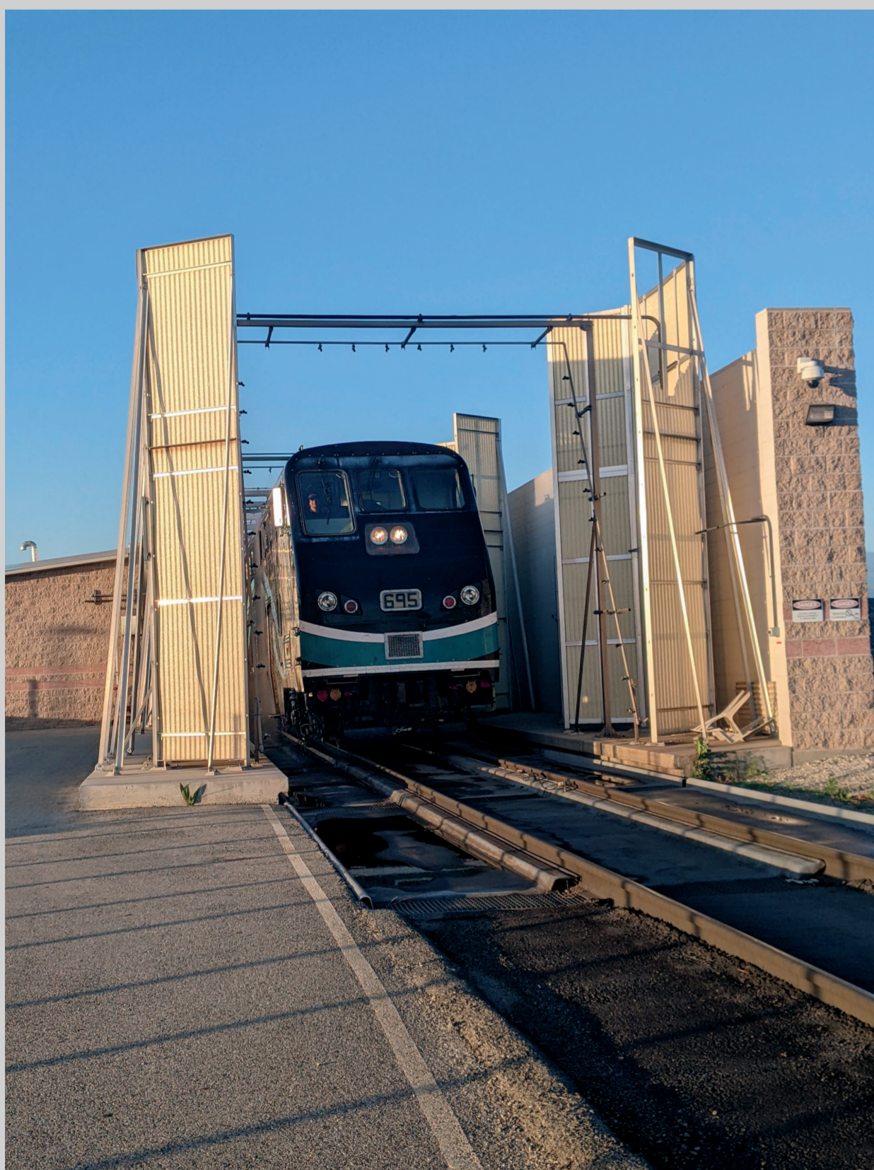
Automated Train Wash
