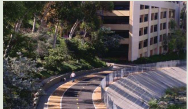
Existing Tracks at Brea Segment
