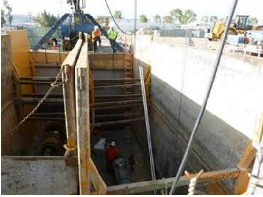
Photo: Jack and bore operation at Atwood Channel
