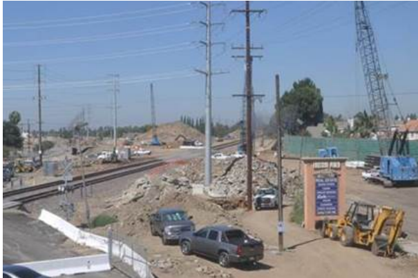
Photo: Looking at Orangethorpe Avenue Crossing
