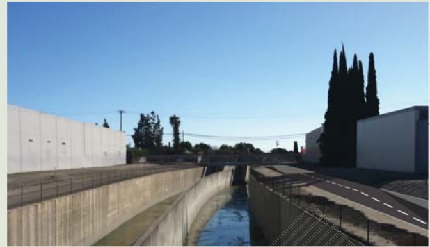
Looking south towards the LOSSAN Rail Corridor from Stage Road with proposed OC Loop Bikeway
